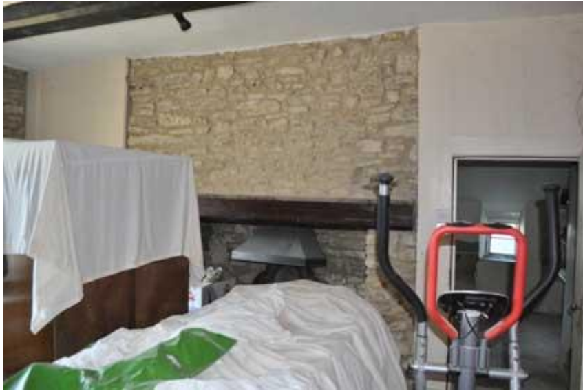
Plate 4 Panelled cupboards either side of fireplace (G3)
