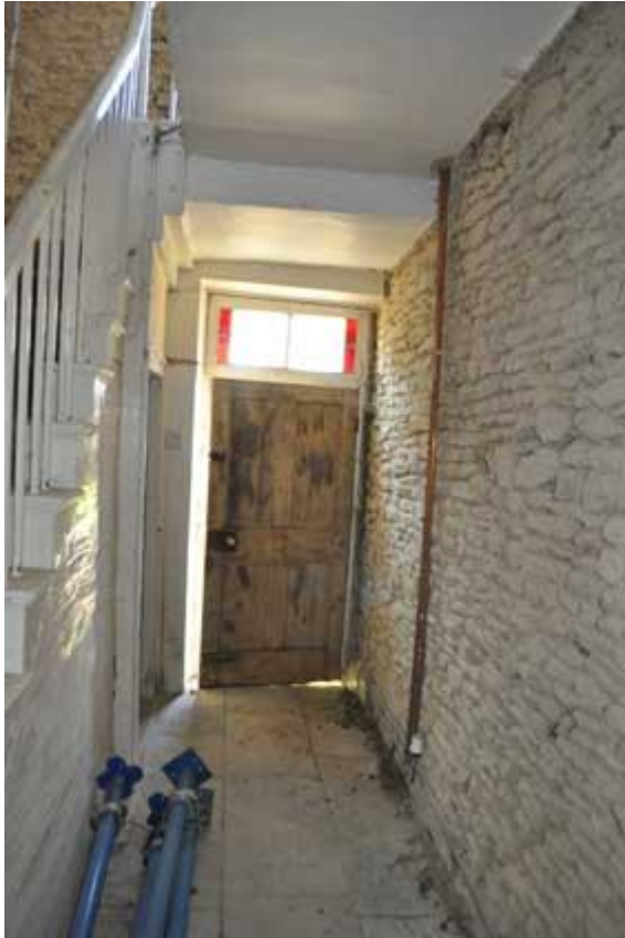
Plate 3 Internal view of front door
