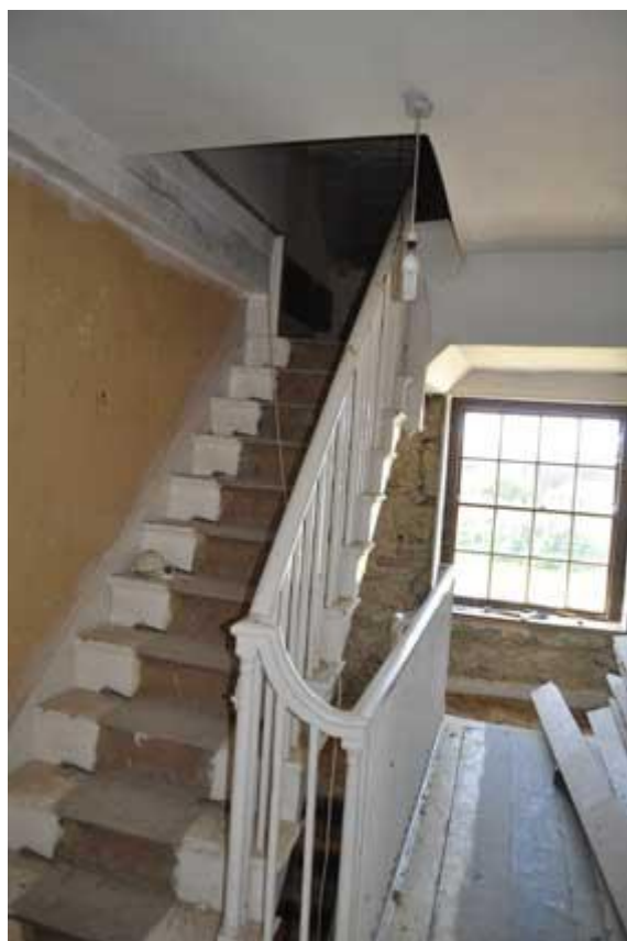
Plate 8 Stairs on landing (F1)
