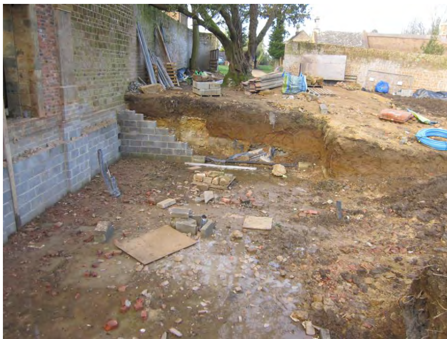
Plate 28: Unmonitored excavation and underpinning
