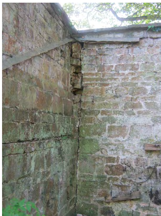
Plate 37: Shed wall butting garden wall
