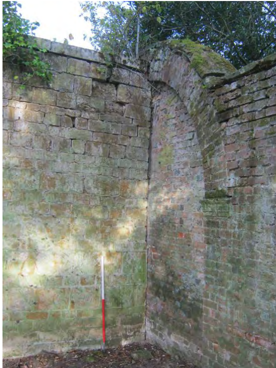
Plate 22: West wall butt joint
