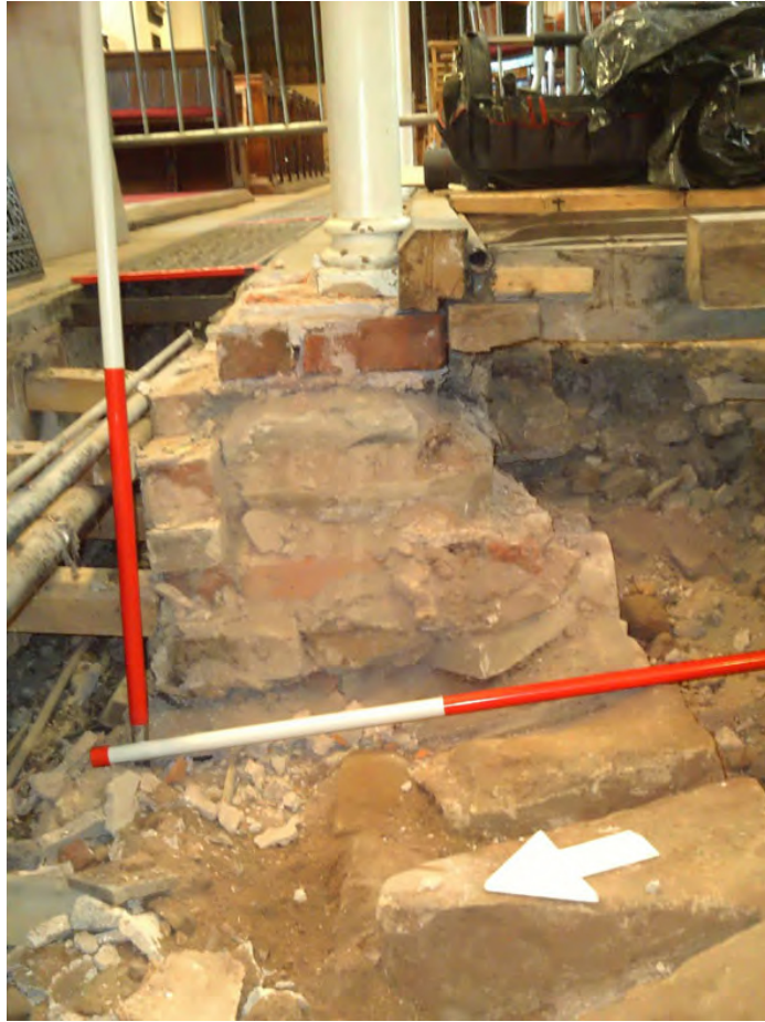
Plate 3. Elevation of Stanchion pad 09
