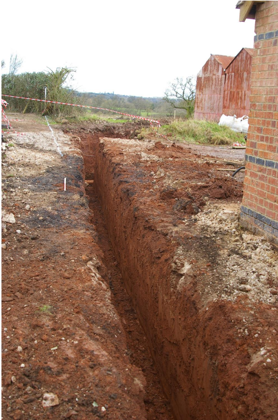
Plate 4. Trench southwest of Bull Pen looking northwest
