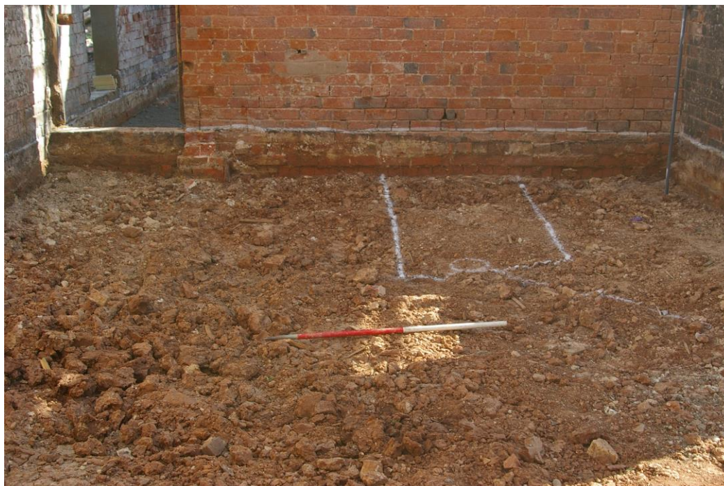
Plate 1. Reduced floor level in Bull Pen looking northeast
