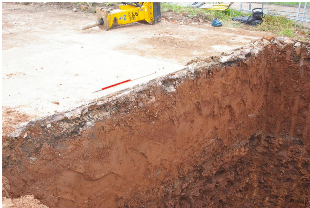
Plate 2. Septic tank trench looking southeast
