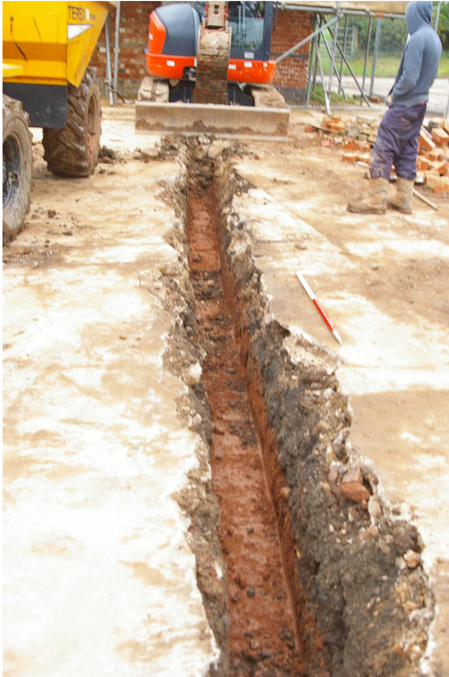
Plate 3. Trench running from Stable Block to septic tank trench looking southeast
