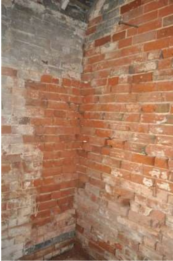
Plate 14: Joint of later northeast elevation of Old Forge
