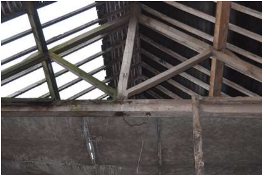
Plate 6: Roof truss in Cow Shed
