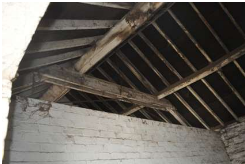
Plate 9: Roof truss in Stable Block
