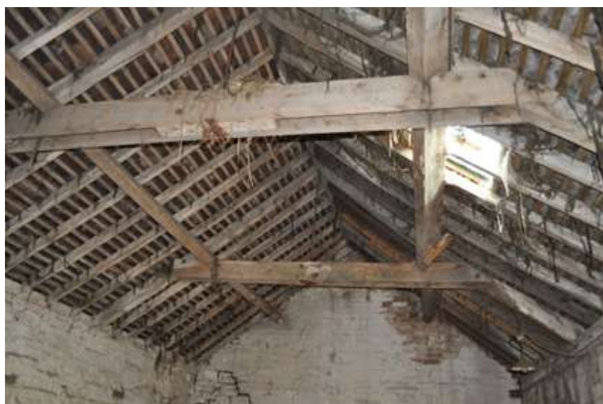
Plate 13: Roof truss in Bull Pen
