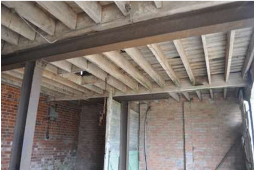
Plate 5: Timber ceiling in Cart Shed
