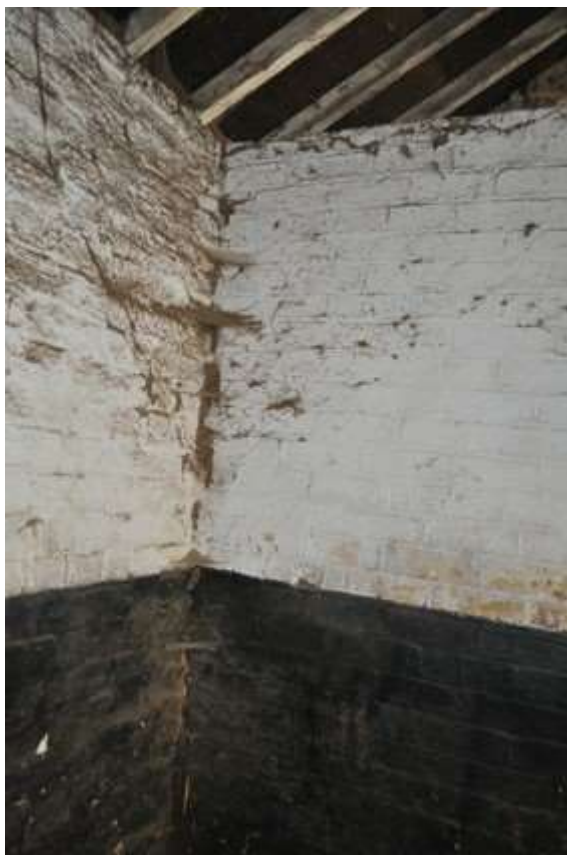
Plate 10: Abutting wall in Stable Block
