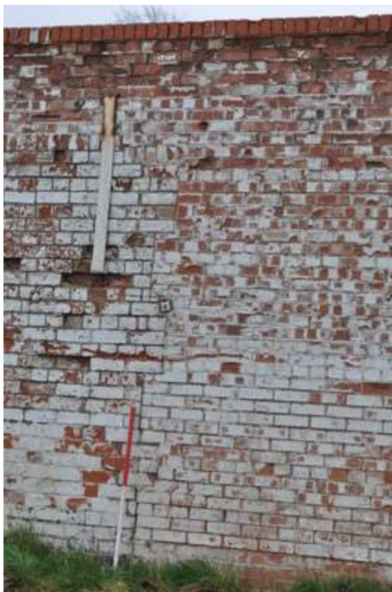
Plate 4: Joint in northeast elevation of Dairy
