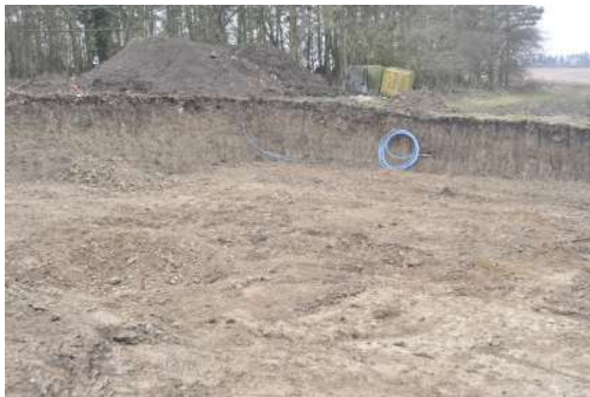
Location of new straw shed. View to southwest.
