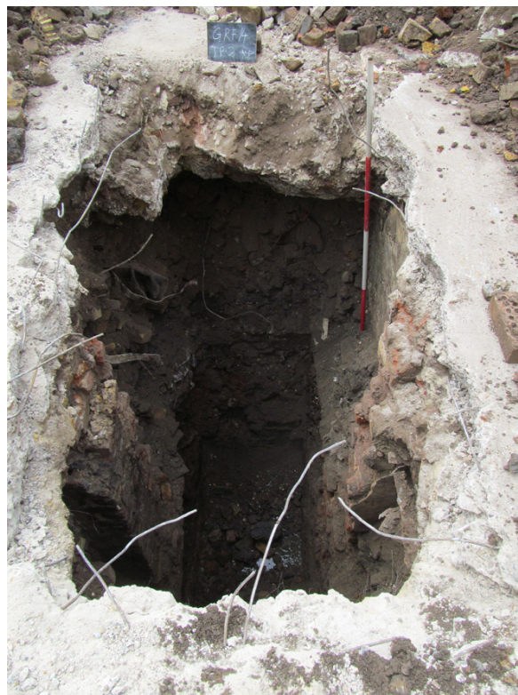
Plate 4: TP.2 – general overview, looking west
