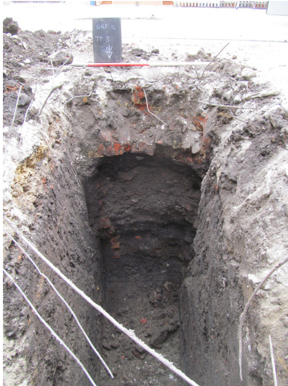
Plate 7: TP.3 – south section, looking south
