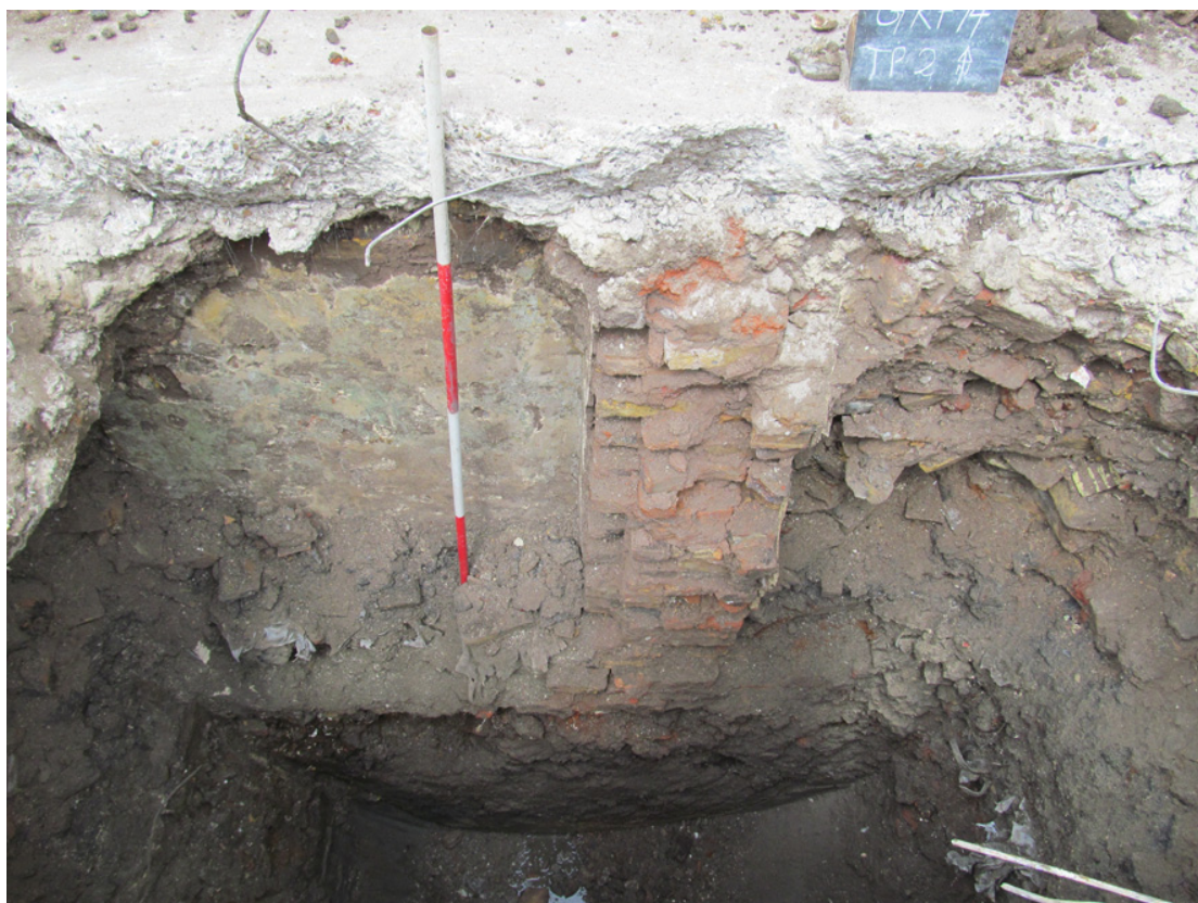
Plate 5: TP.2 – north section, looking north
