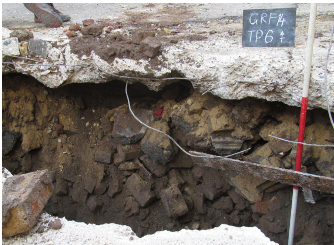
Plate 14: TP.6 – north section, showing brick wall underneath the concrete surface, looking north
