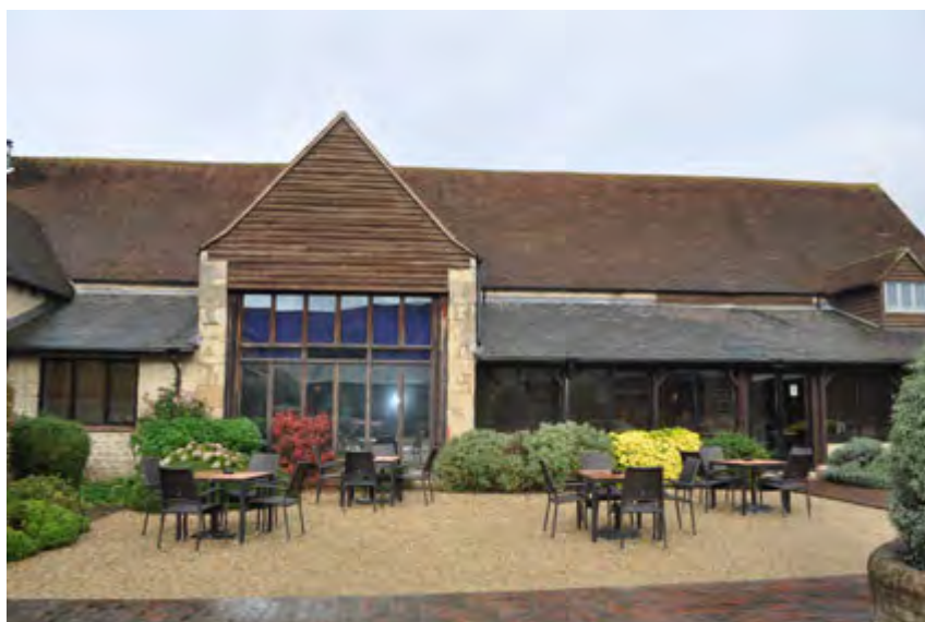
Plate 8: South elevation of Chapel / Barn
