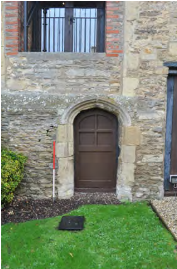
Plate 6: 15 th century doorway
