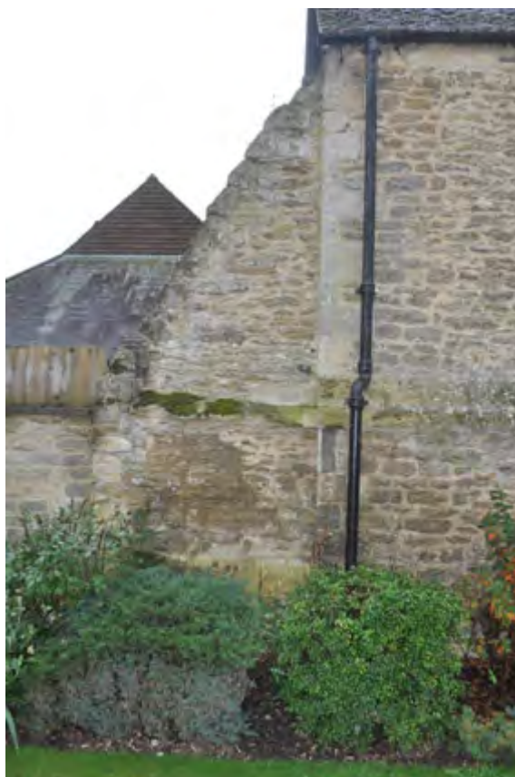
Plate 7: 13 th century angle buttress
