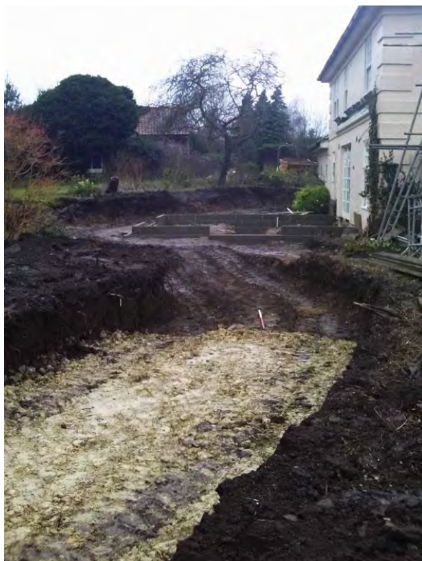
Plate 1. Excavated driveway/ path to Pool/Gym Room. West view.
