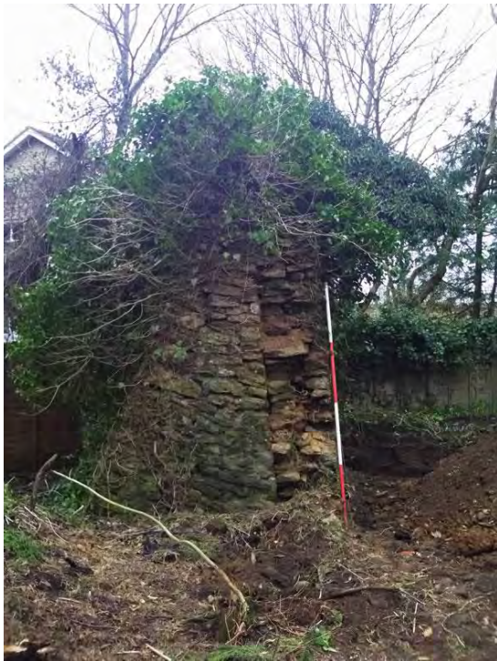
Plate 3. North section of wall 11 and butress. South view
