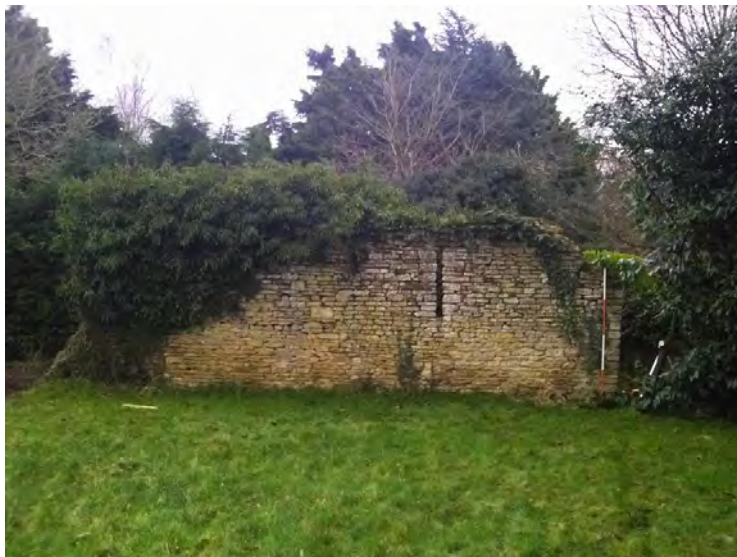
Plate 5. West face of Wall 9.
