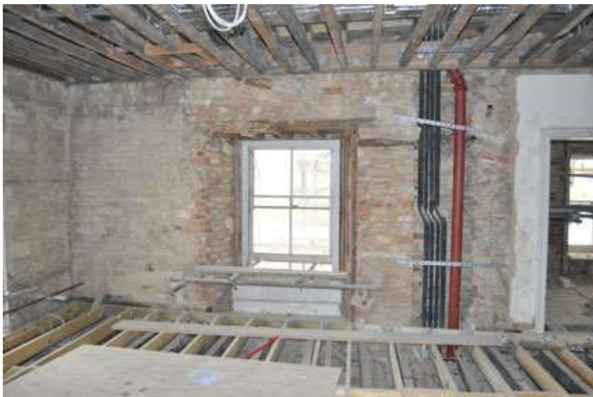
Plate 35: Window inserted in E wall room S7
