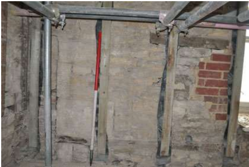
Plate 37: Butt joint in E wall of S8
