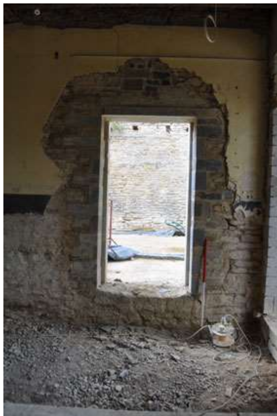
Plate 20: Inserted door G23
