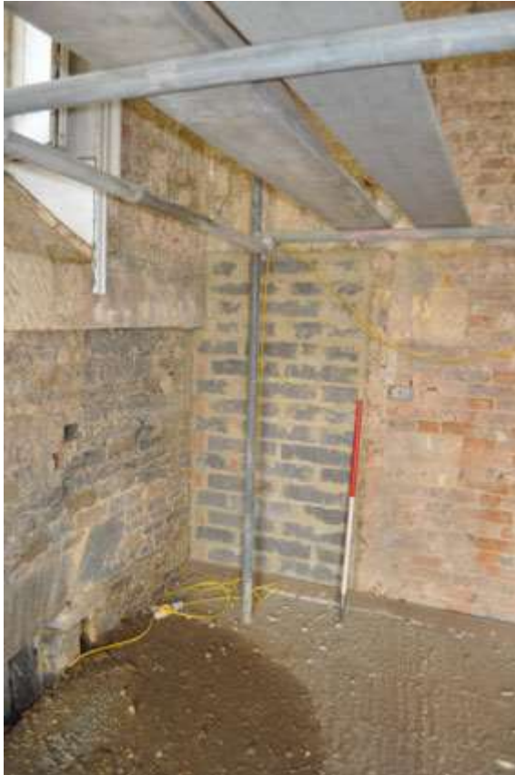
Plate 16: Blocked doorway G4
