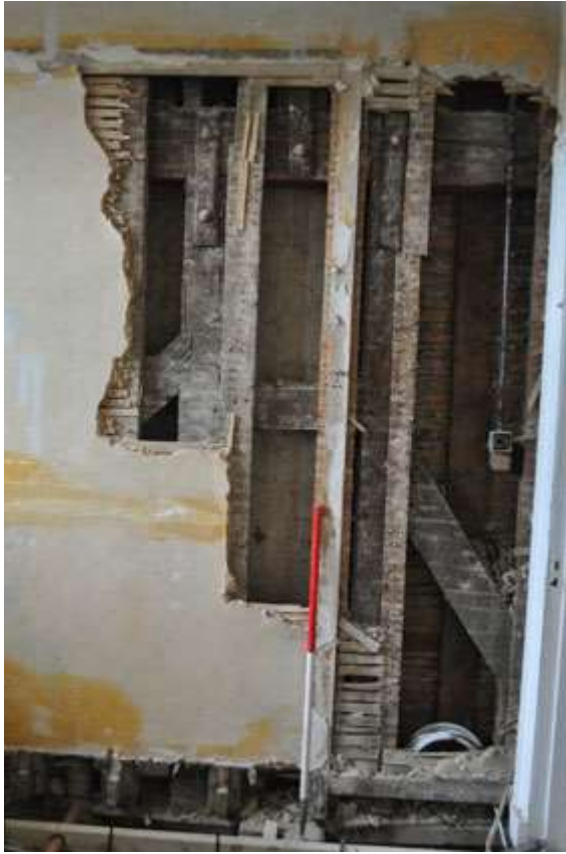
Plate 23: Timber framing F2
