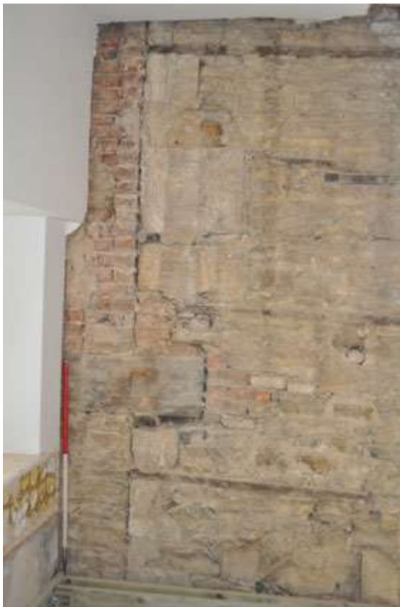
Plate 26: Butt joint in E wall F13
