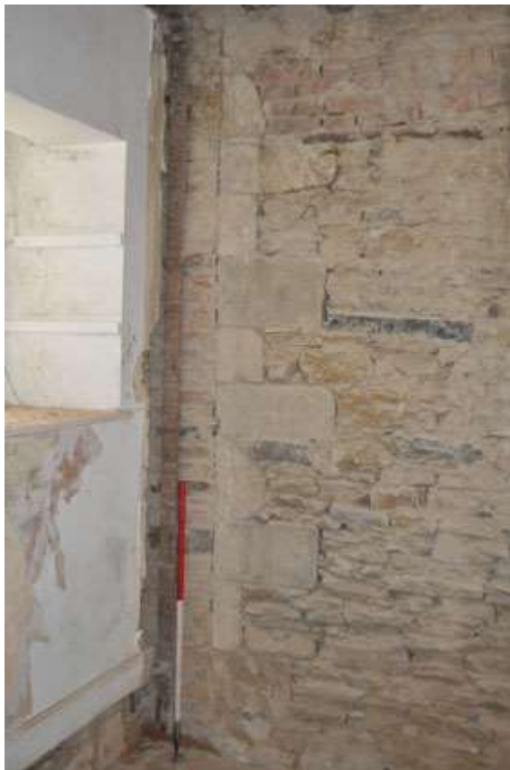
Plate 7: G15 butt joint in E wall
