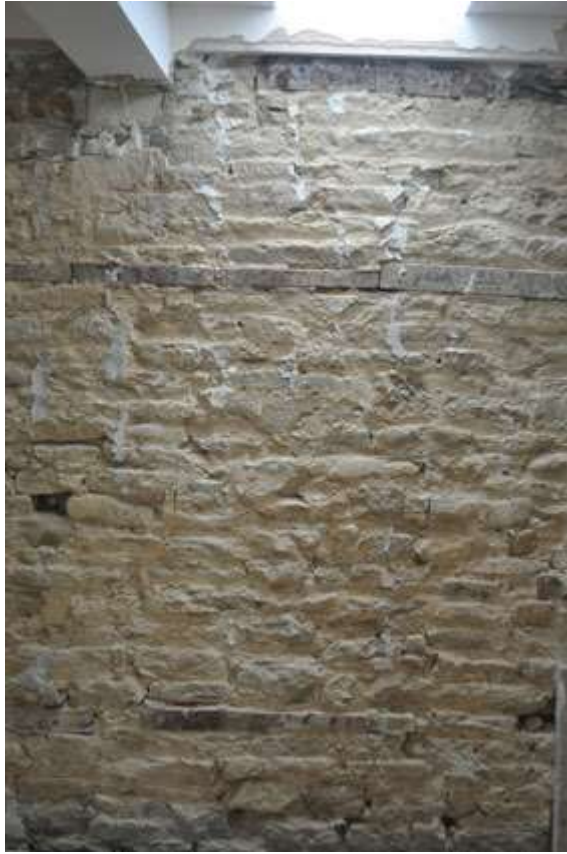
Plate 29: Rubble wall N wing first floor
