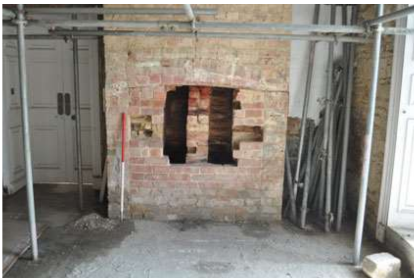
Plate 15: Fireplace and chimneybreast G3
