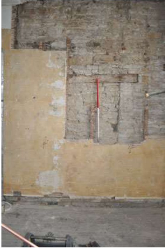
Plate 21: Timber lintel and doorway F5
