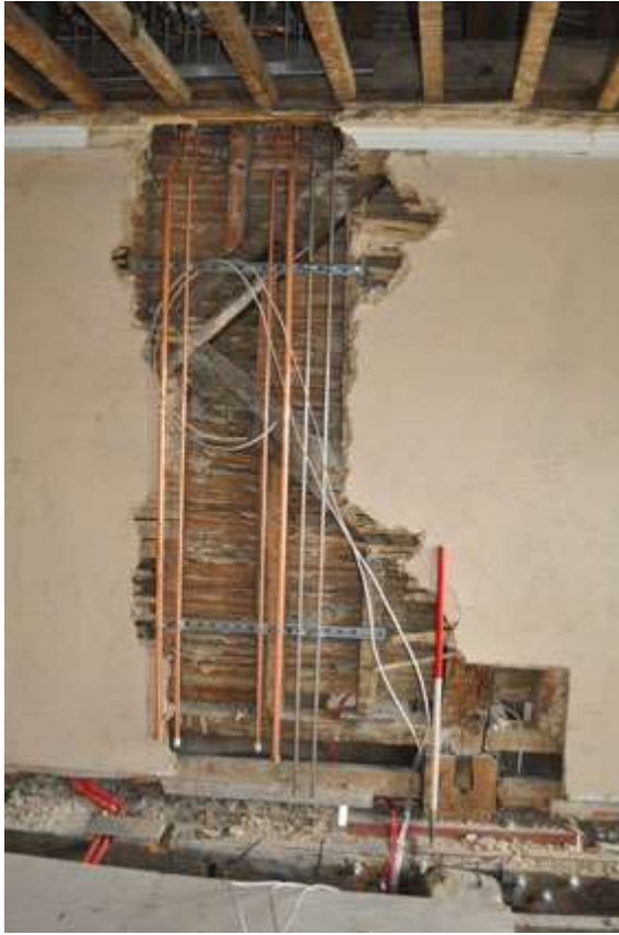
Plate 41: Timber framing S13
