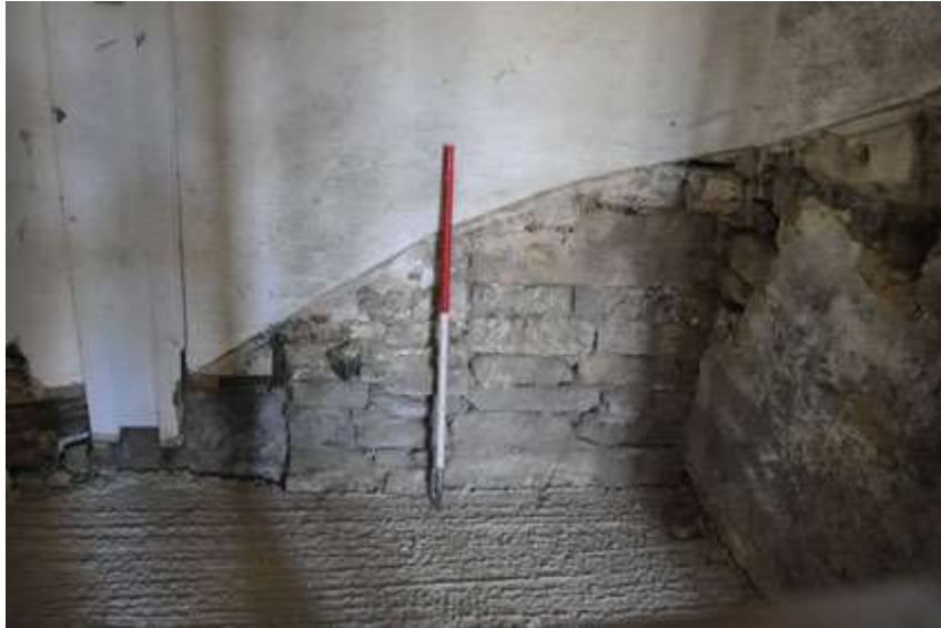
Plate 12: Butt joints G10
