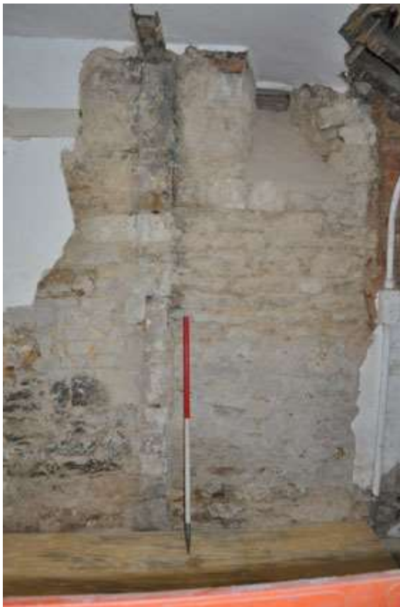
Plate 11: Wall with butt joint G8 / G9
