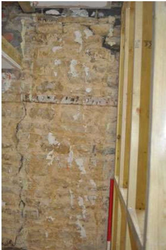
Plate 30: Rubble wall N wing first floor
