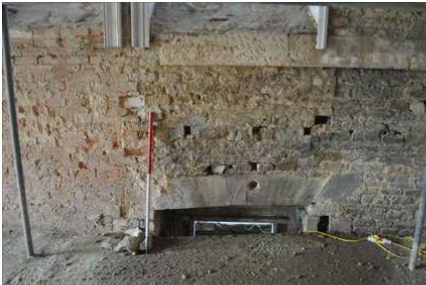
Plate 17: Butt in wall G4
