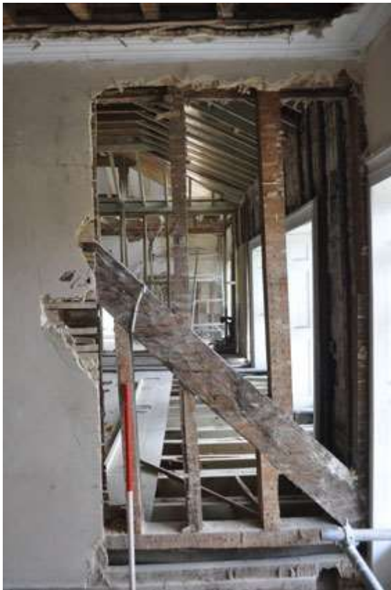
Plate 42: Timber framing S13
