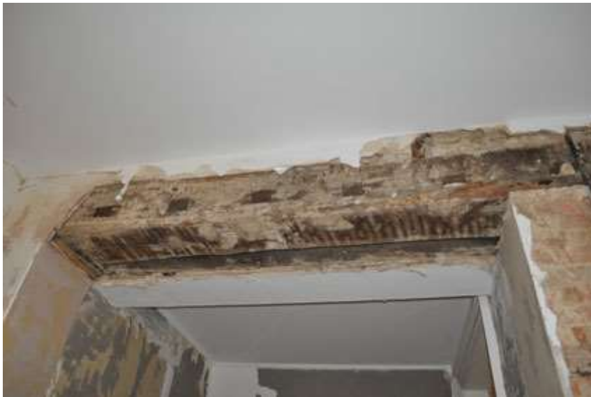
Plate 9: Timber beam supporting wall above G14 / G15
