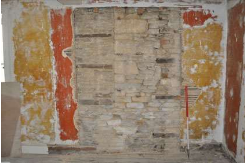
Plate 10: Remains of blocked window in N wall G13
