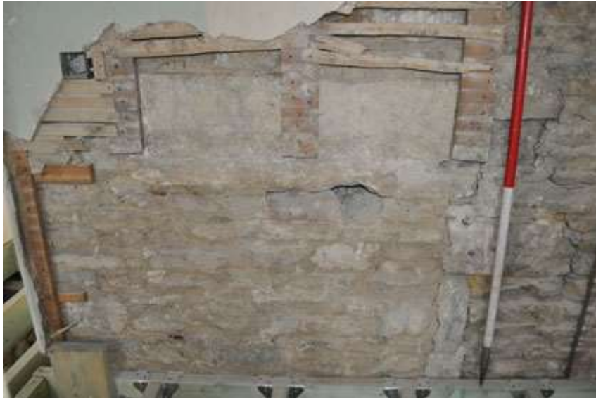
Plate 25: Blocked up fireplace
