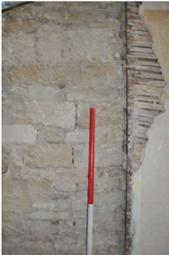
Plate 22: Butt joint in wall F5
