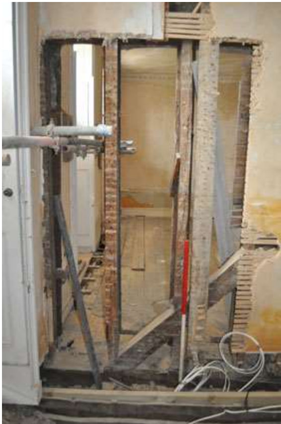
Plate 24: Timber framing F2
