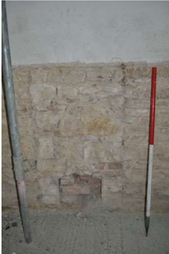
Plate 14: Blocked feature in S wall of G17
