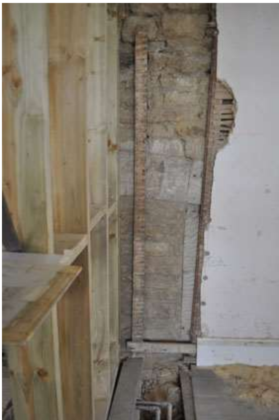
Plate 5: Blocked fireplace G16
