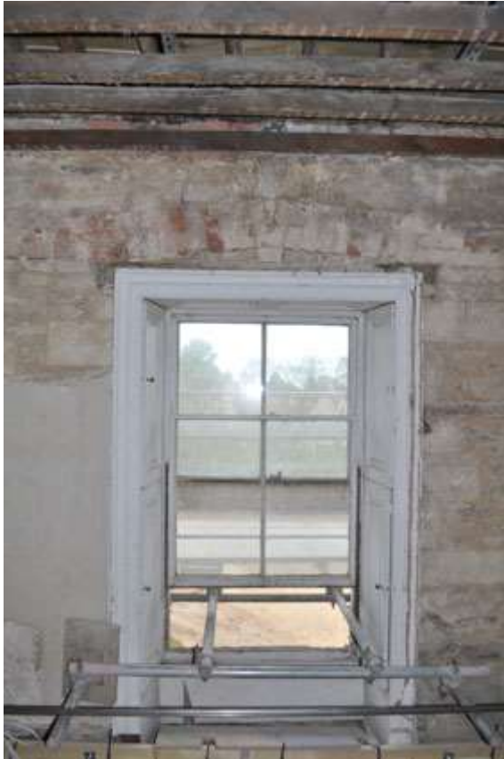
Plate 34: Window in situ with brick arch S6
