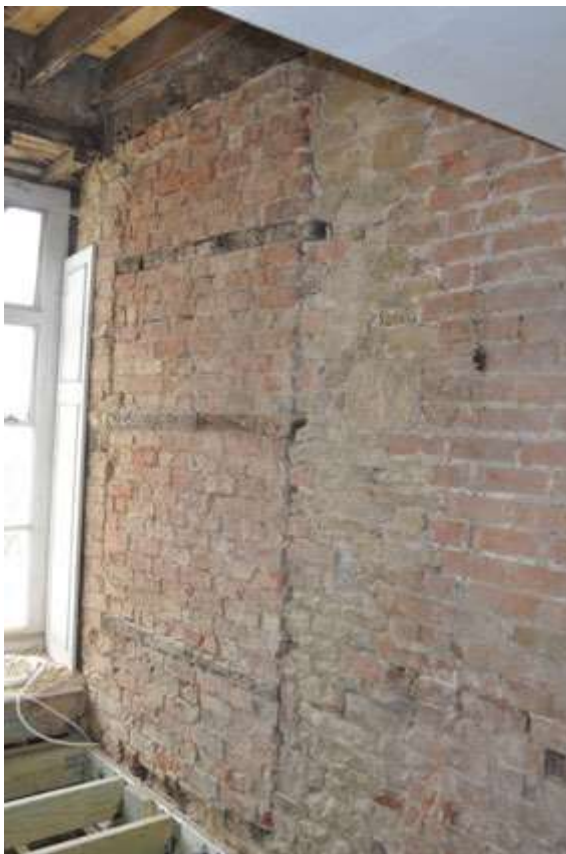
Plate 28: Blocked doorway F14
