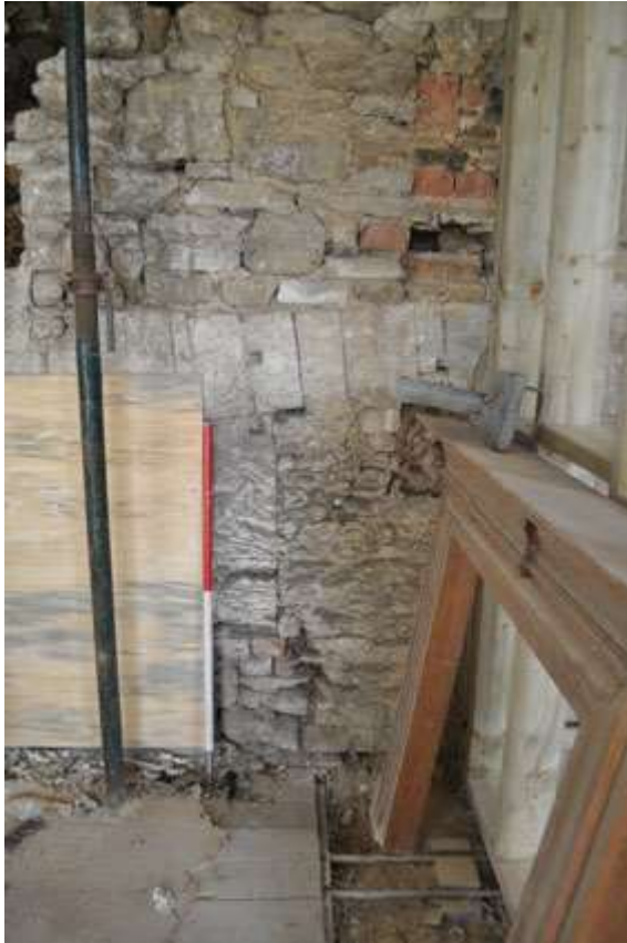
Plate 4: Blocked fireplace G1
