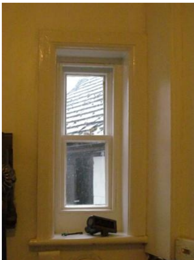
Plate 6: Sash window in east elevation
