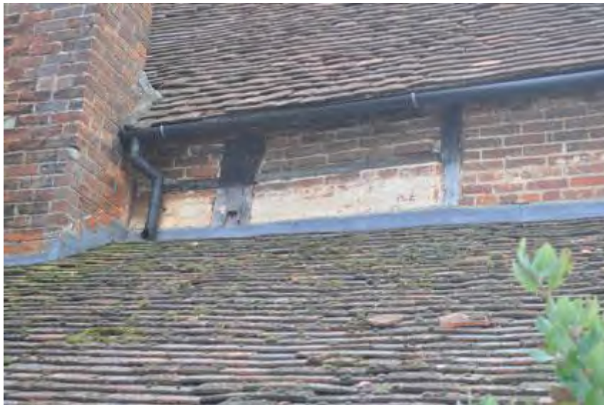
Plate 27: Timber framing with remains of jowl post
