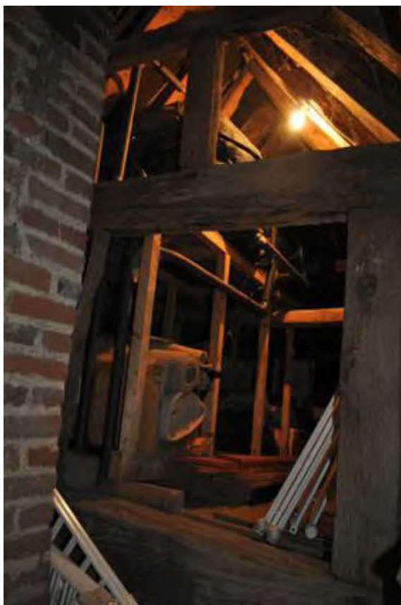
Plate 26: Truss in attic
