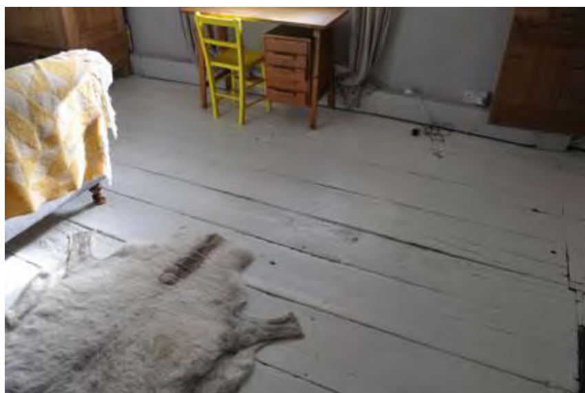
Plate 18: Wide floorboards room F2
