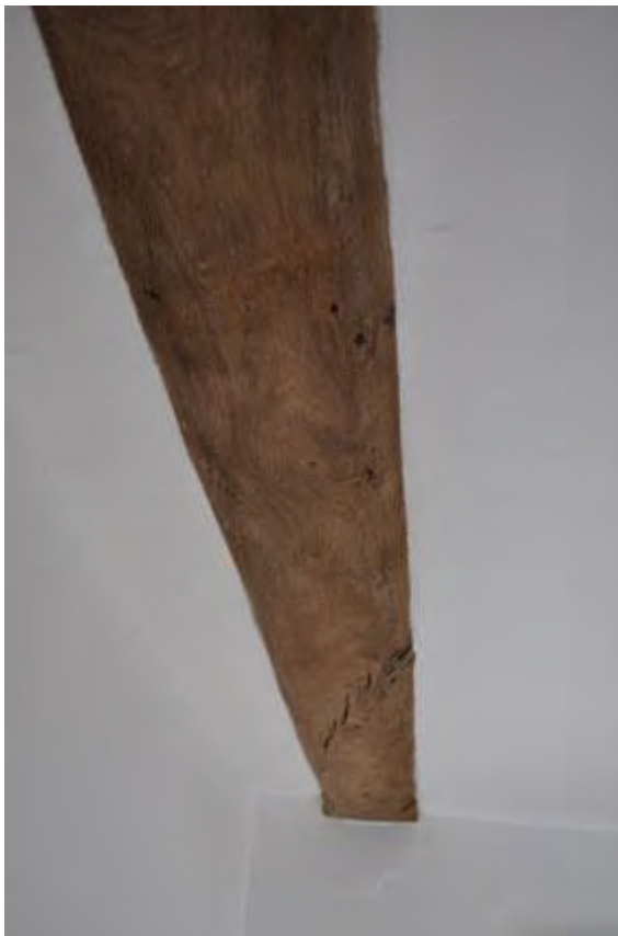
Plate 24: Chamfered beam room F8
