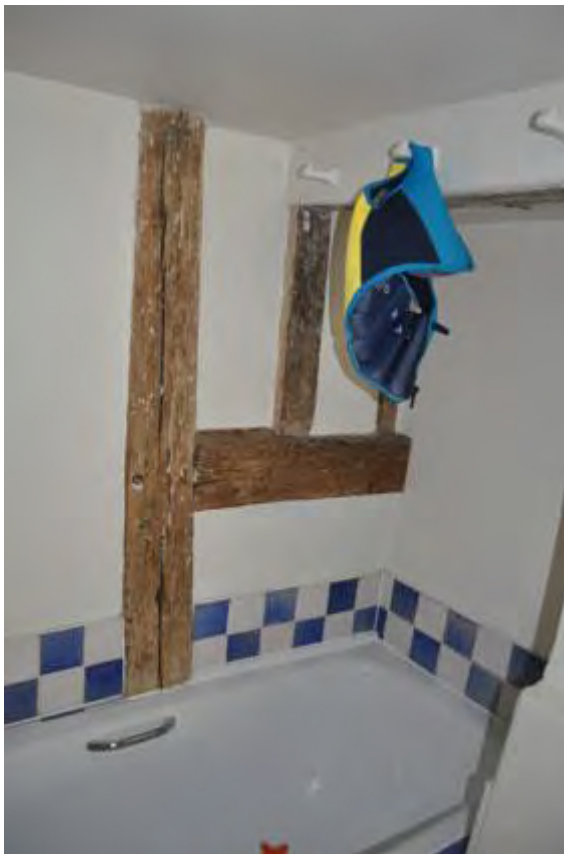
Plate 20: Timber framing room F3
