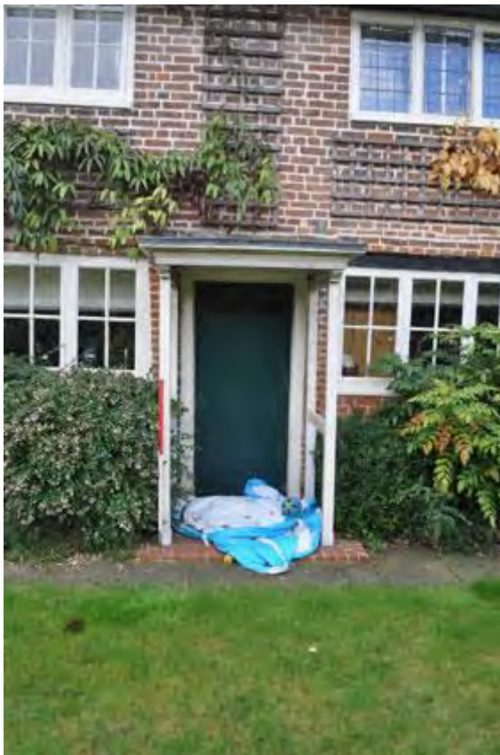
Plate 2: Porch on the northeast façade
