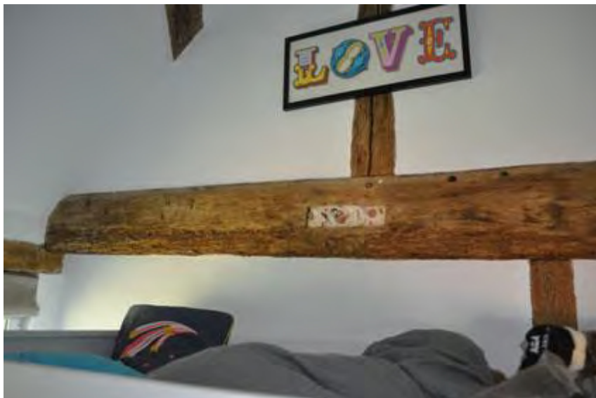
Plate 21: Part of truss room F4
