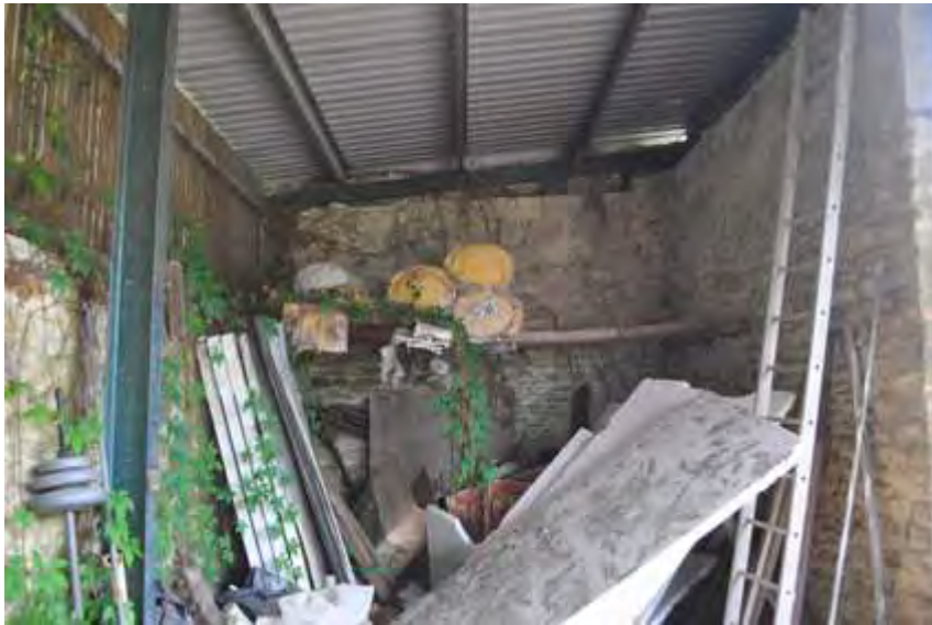
Plate 4: Interior of east end of eastern building
