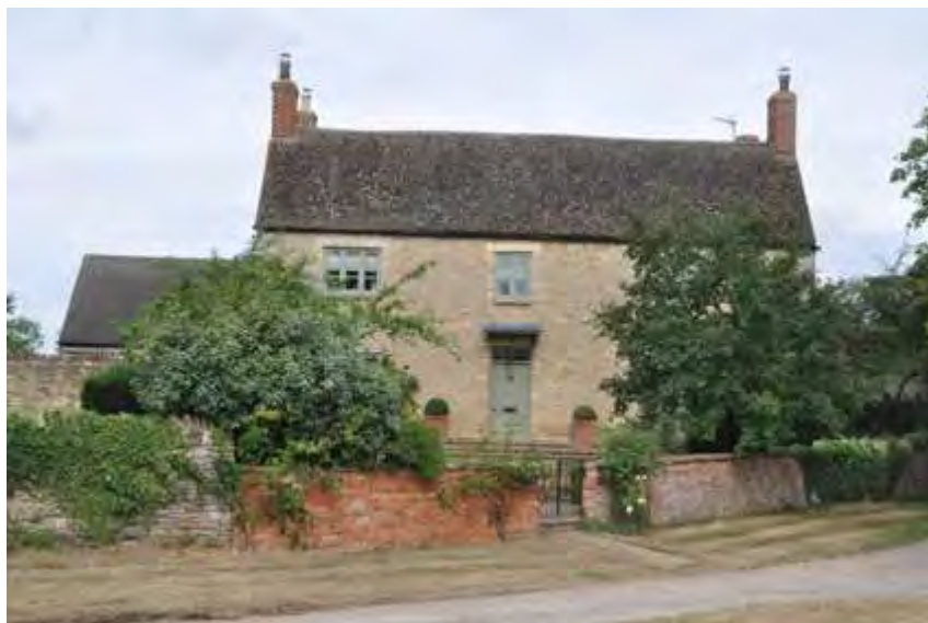
Plate 6: Front of Manor Farm
