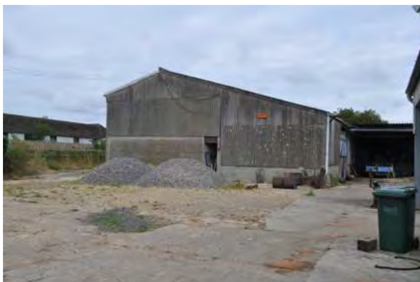
Plate 2: Corrugated sheet and cinder block building
