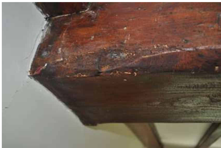
Plate 7: Chamfered ceiling beam, west end
