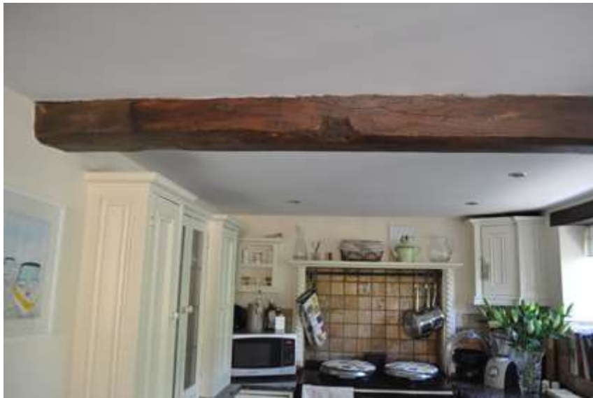
Plate 5: Ceiling beam in kitchen
