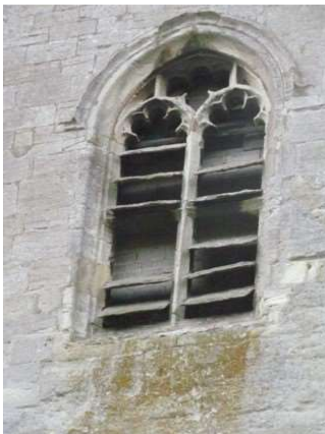
Plate 8: North window in bell tower
