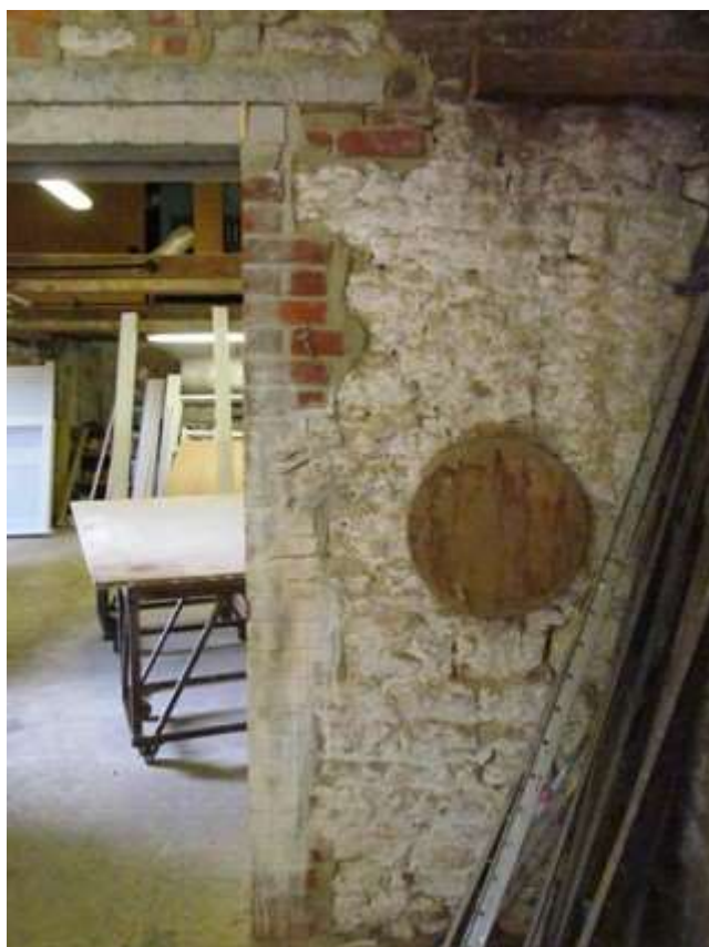
Plate 2: Lining of passage between building 4 and 5
