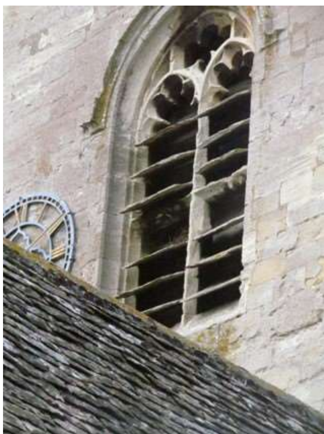
Plate 9: East window in bell tower
