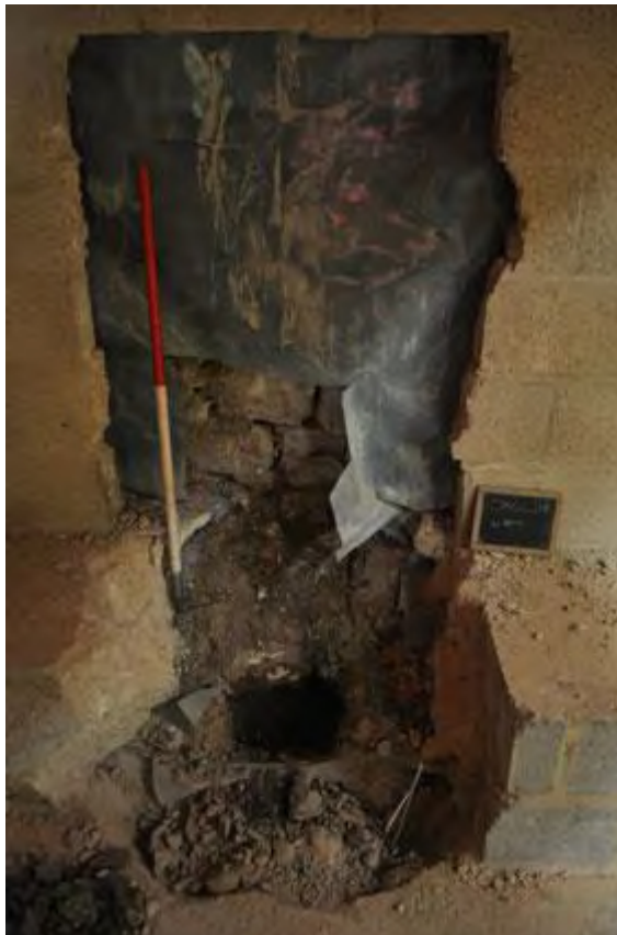
Plate 2: East wall wider foundation 45
