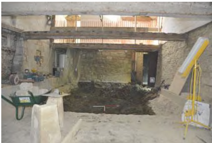
Plate 5: Wall 48/76 at the south end of north part of the barn
