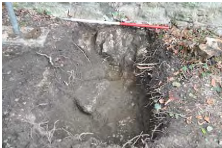
Plate 1: Wall 3 and buttress foundation 4
