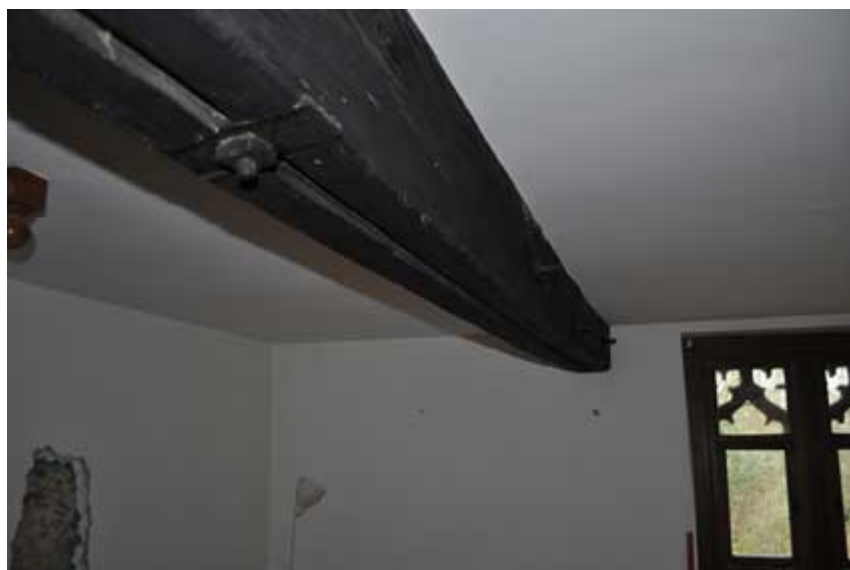
Plate 4 Beams in lower floor south unit
