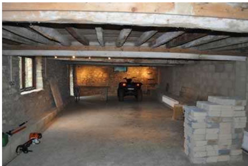
Plate 5 Lower level of barn or undercroft
