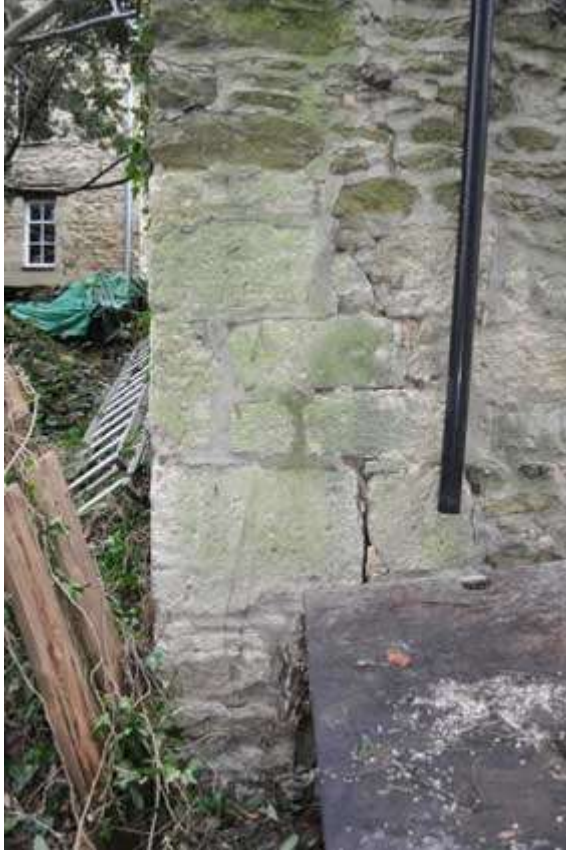
Plate 8 No indication of vertical butt, but three bandings of stone
