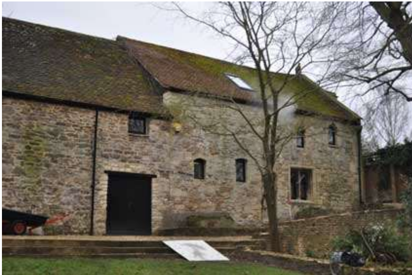
Plate 9 No indication of butt joint at the south end
