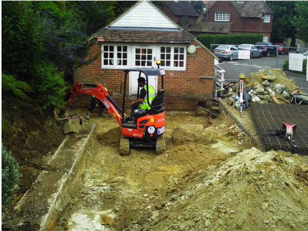
Plate 1 SE view of the open trench during groundworks
