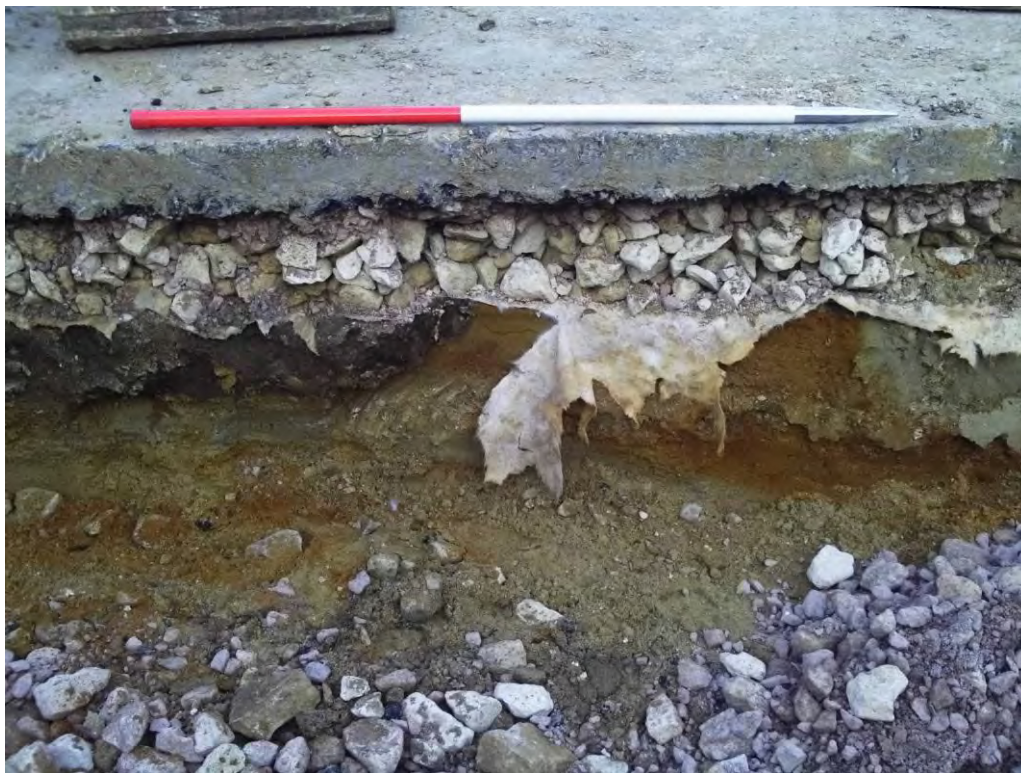
Plate 2 NE facing representative section of the excavation area
