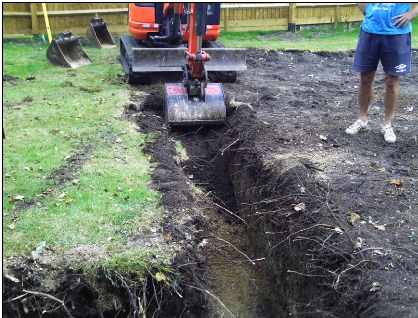
Plate 1: NNE view of NW corner of Area A footings working shot
