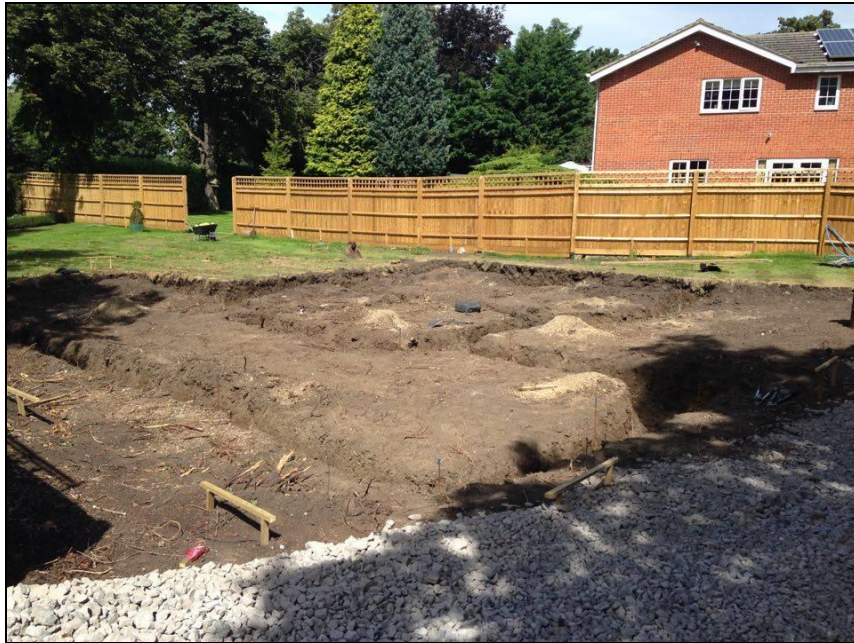
Plate 2: Completed excavation of footings in Area A. NW facing
