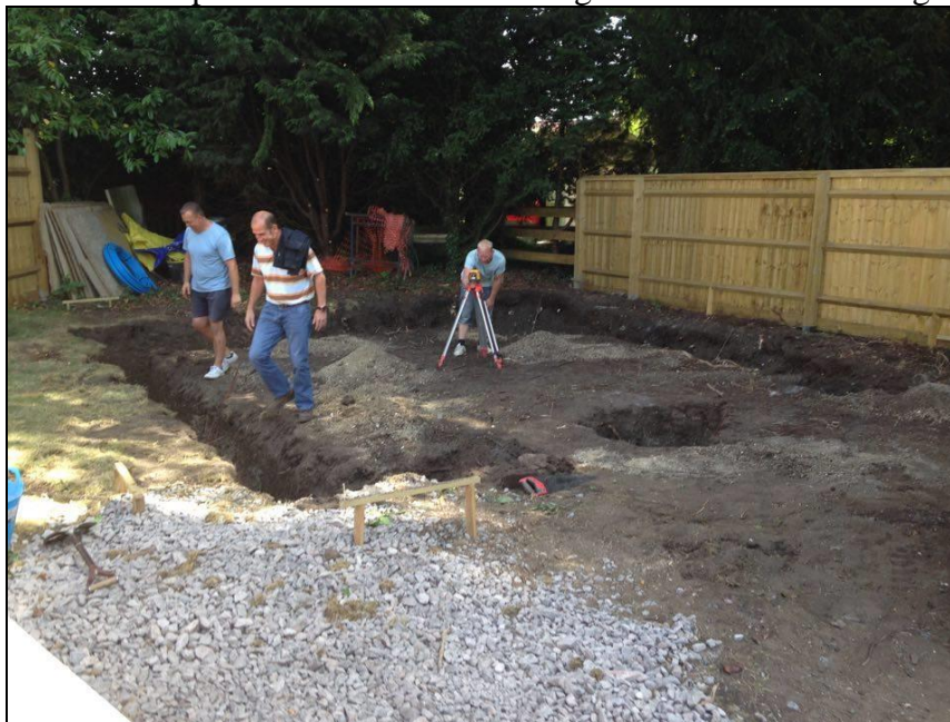
Plate 3: Completed excavation of Area B. East facing
