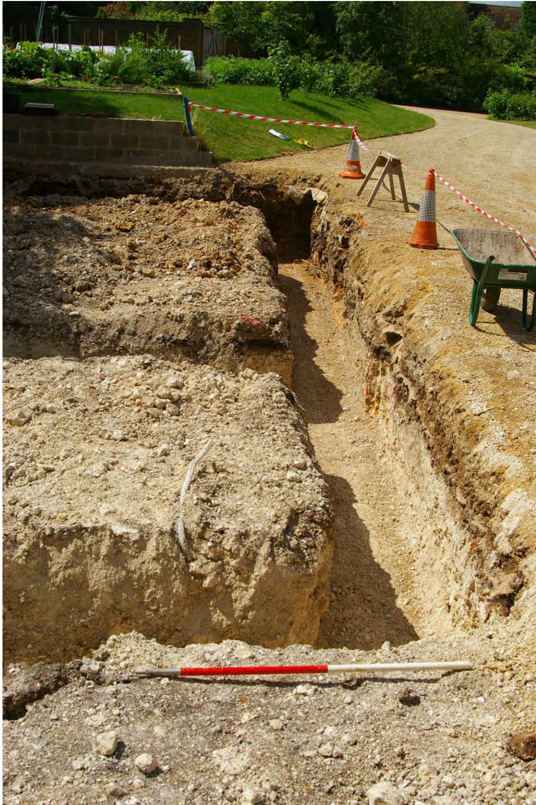
Plate 2. General shot of foundation trench looking west
