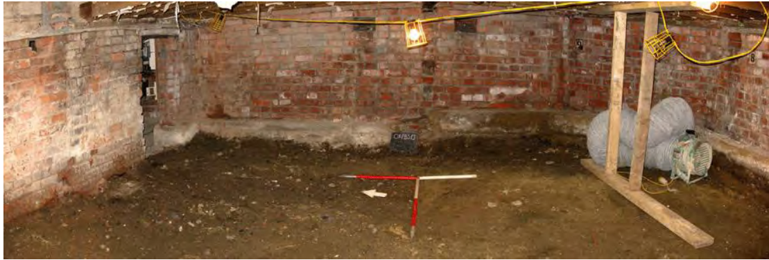
Plate 6: Deposit (101), after initial ground reduction and internal walls demolition, looking east
