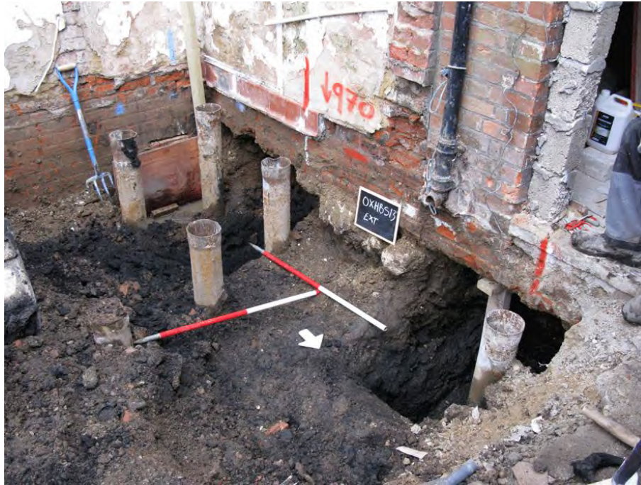
Plate 2: Deposit (105) during ground reduction within the courtyard, looking southwest
