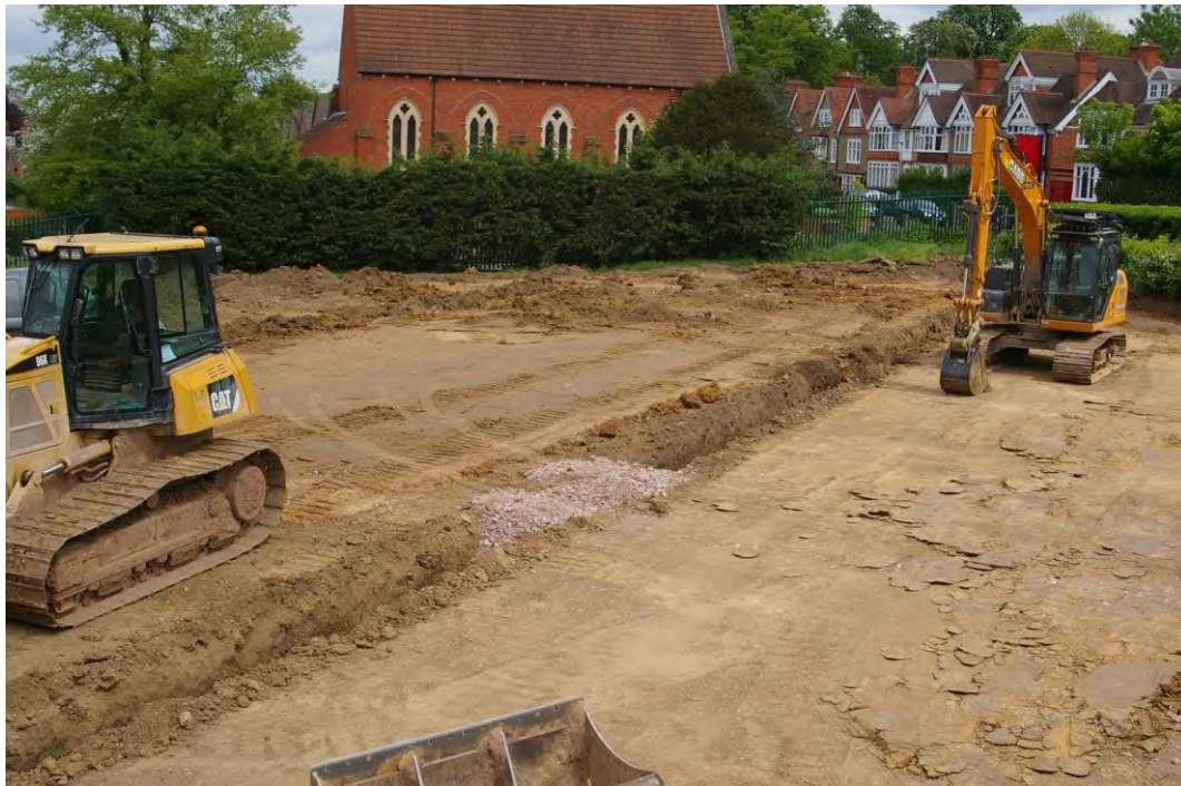
Plate 2. General view of site looking southeast
