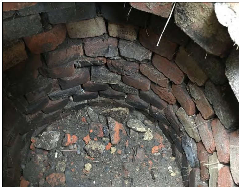
Plate 2: Internal view of soakaway shaft.
