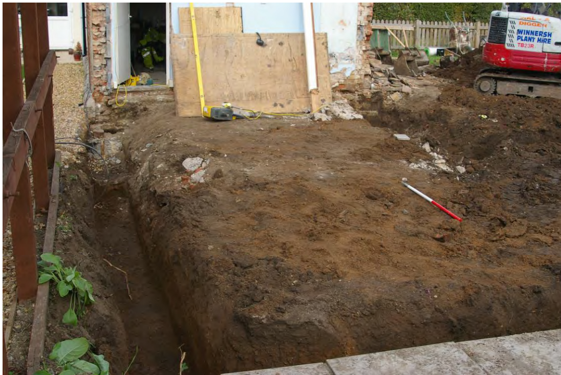
Plate 1. Foundation trench looking north
