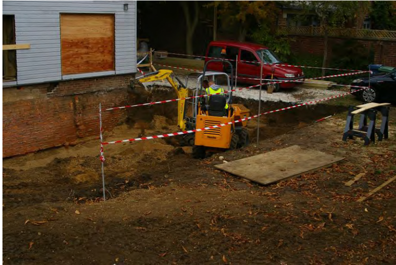
Plate 1. Working shot of basement excavation
