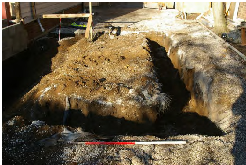
Plate 2. Foundation trench on eastern side of building
