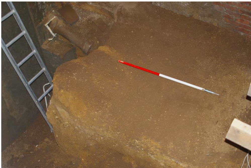
Plate 2. Excavations in the rear cellar
