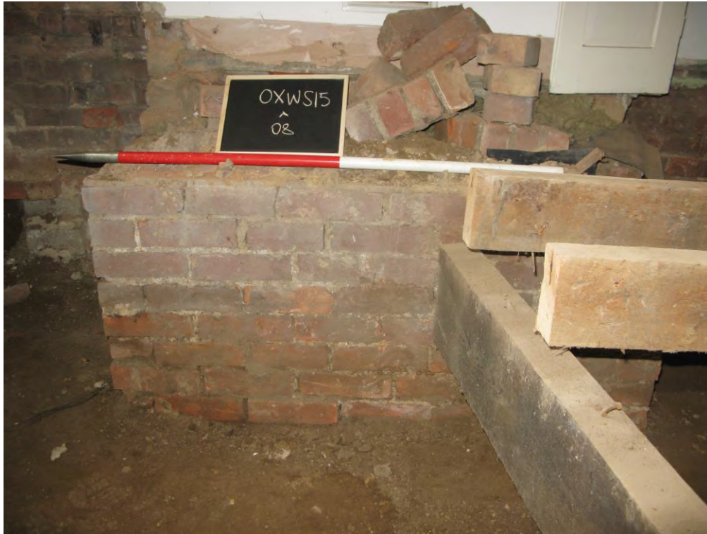
Plate 1. Chimney foundation 08
