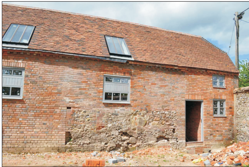
Plate 1. The rubble and brick wall of the Phase 1 building.
