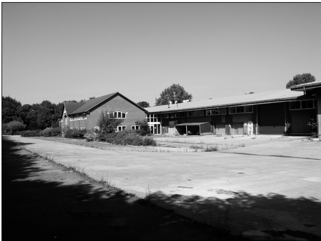
Figure 2. A view of the site, looking from the southeast corner towards northwest.
