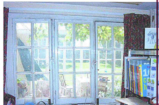
Plate 7: Casement Window Interior View
