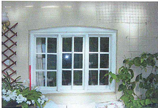
Plate 6: Casement Window Exterior View
