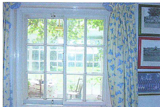
Plate 3: Horizontal Sliding Sash Interior View
