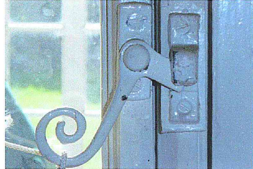
Plate 5: Cockspur Catch Detail
