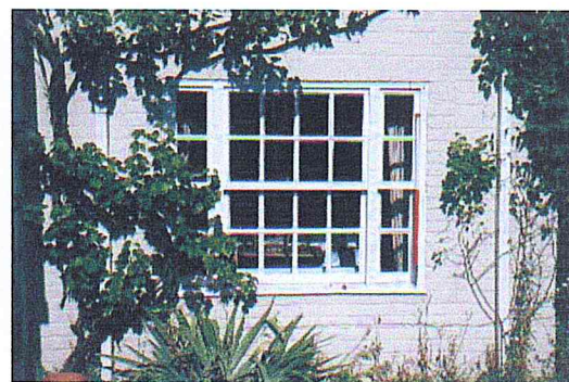
Plate 12: The tripartite window in the rear elevation of the two-storey extension
