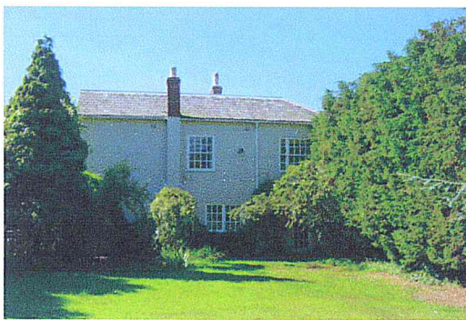
Plate 11: The assortment of windows in the eastern elevation of the extension
