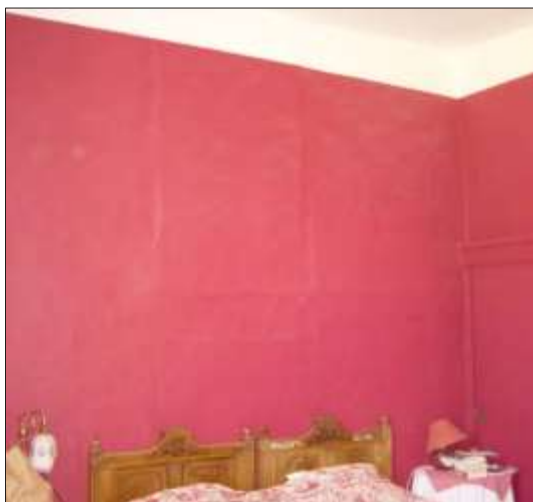
Plate 3: Ghosts of timber construction visible through Wall finish.
