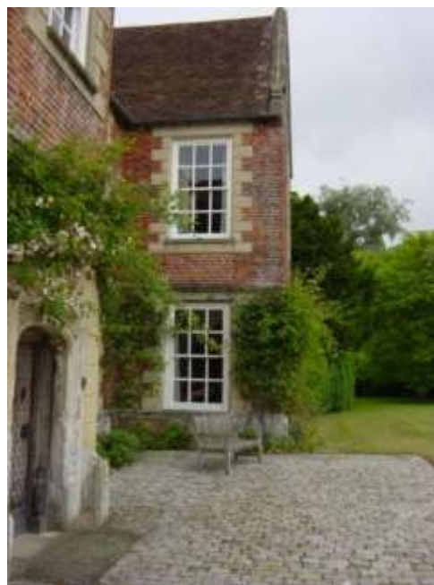
Plate 2: Re-instated upper window as part of the 1980s alterations
