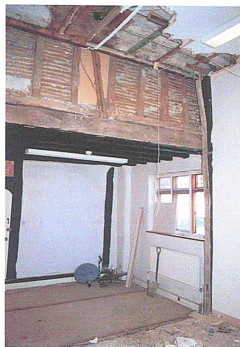
Fig 4 (clockwise) Frame B showing the corner post reversed with the jowled head facing inwards The junction of frame B (left) & frame A (right); frame B is rebated for a door Frames B (foreground) & A looking west; 16 th century doors in the background Post of frame B looking north; lath and plaster infilling frame A at first floor level behind Frames A (foreground) & B looking east
