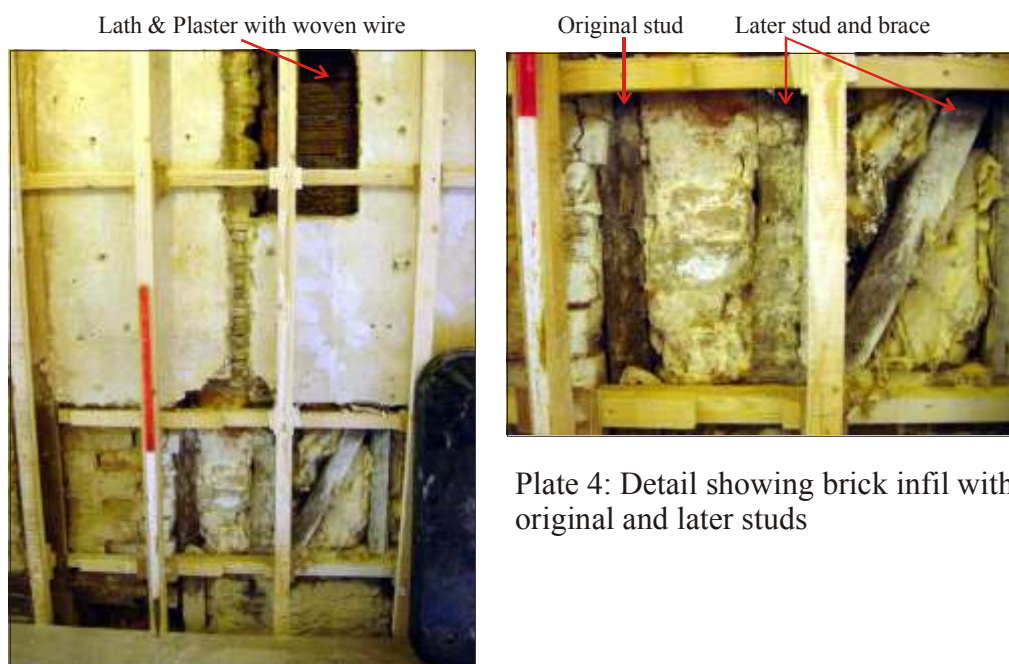
Plate 3: The different materials used in re-building/ repairing the Ship Street Front at ground floor level
