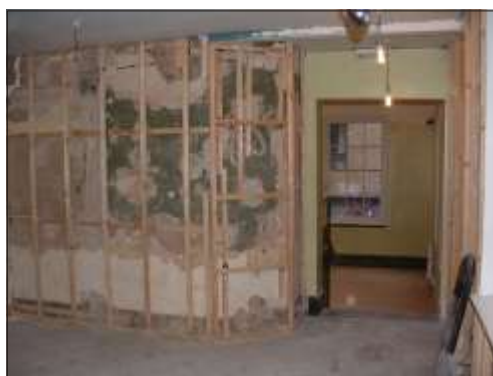
Plate 7: Chamfer on chimney breast and access to front room
