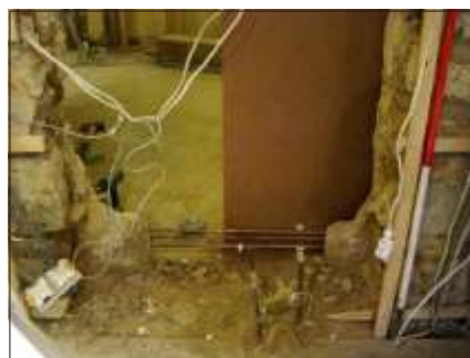
Plate 6: Detail of Breach
