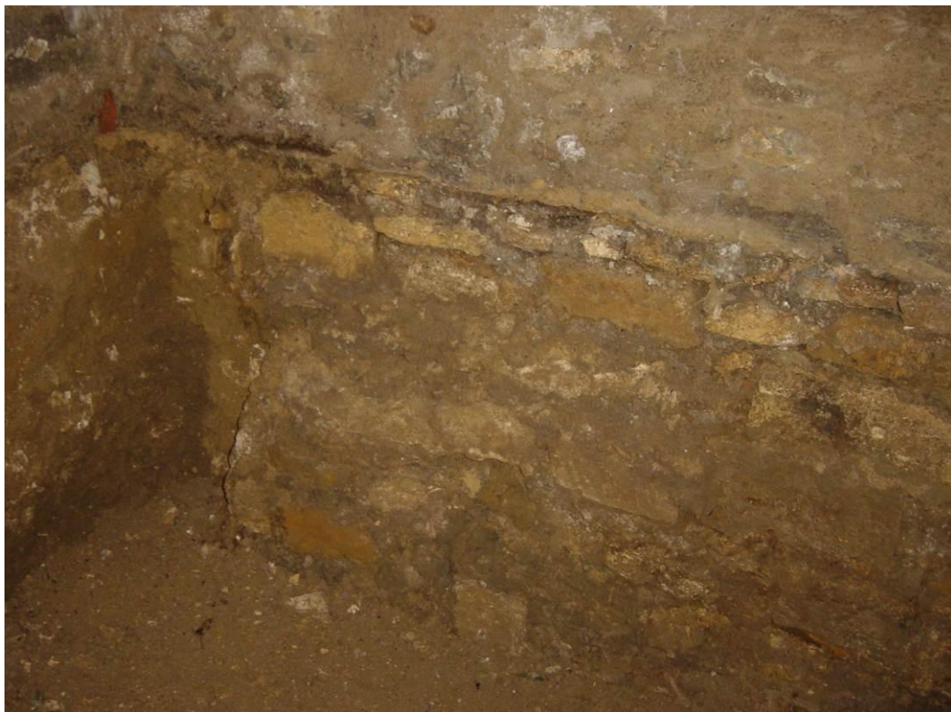
Plate 18. The sloping earlier footings of the northern wall of the 'Wood Shed', Trench 17, possibly part of a bastion on the medieval city wall
