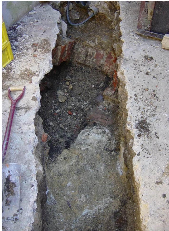
Plate 17. Brick barrel-vaulted drain 816, Trench 22A
