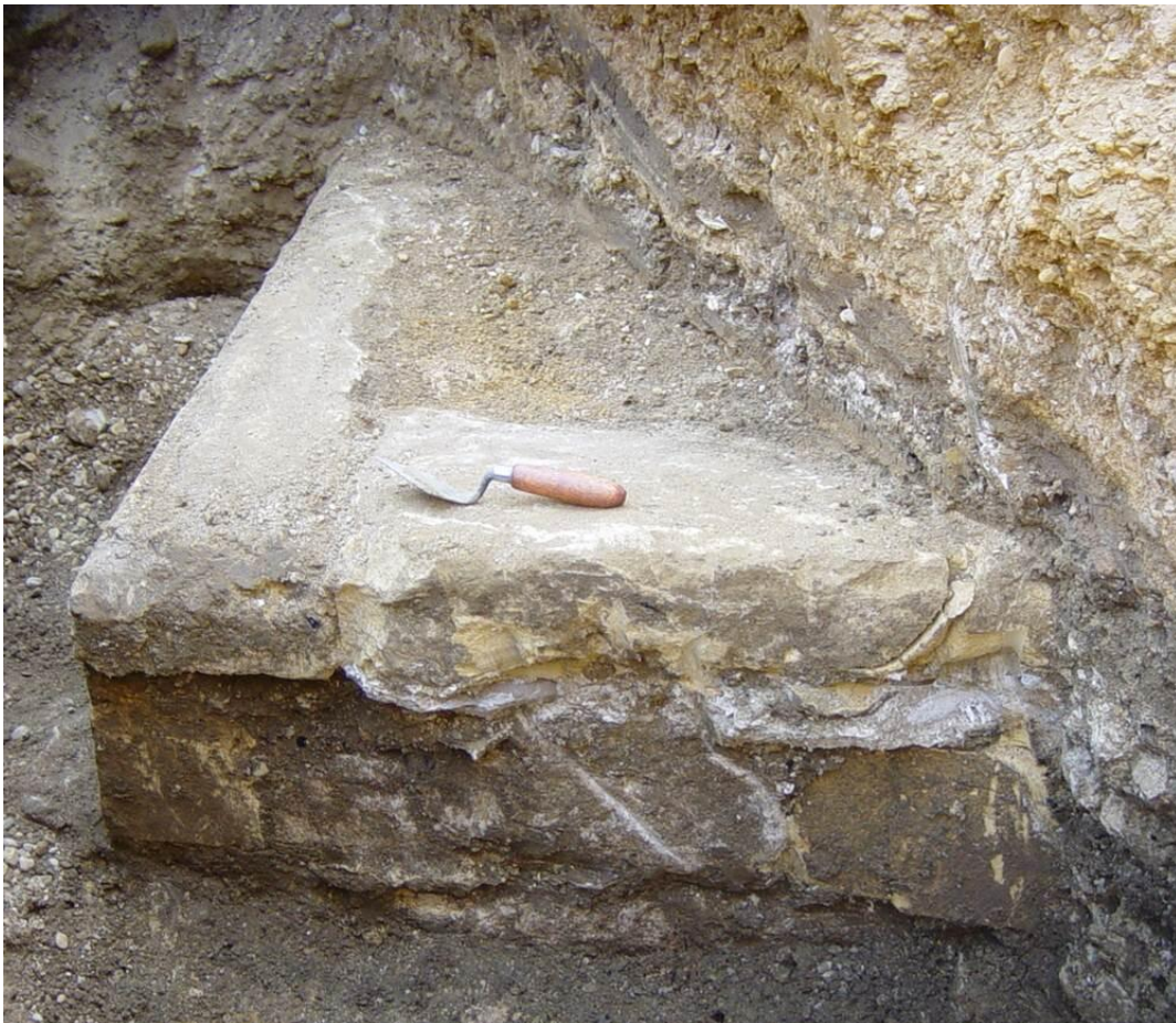
Plate 14. Buttress 714, Trench 10, probably part of the porch entrance into the chapel of Canterbury College
