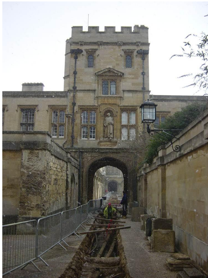
Plate 20. Work in progress at Fell Tower
