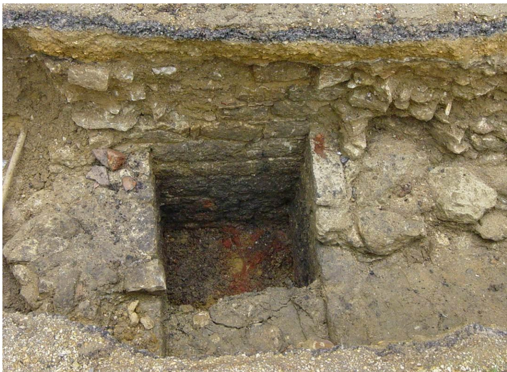
Plate 12. The junction of walls 489, 490 and 491 forming a stone-lined garderobe, with deposit (496) under excavation, Building 7B, Trench 7
