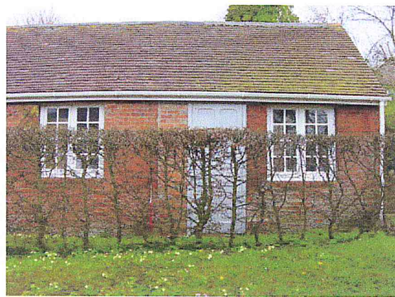
Plate 4: The west elevations showing brick infill in reduced doorway.
