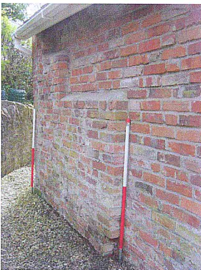
Plate 5: The southern end of the east elevation showing blocked former doorway and window locations
