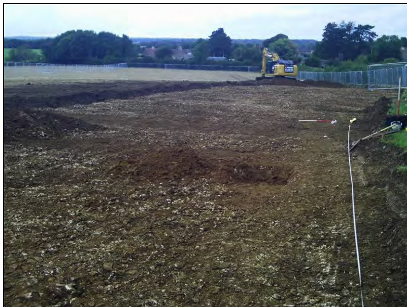
Plate 2: General working shot of the stripping facing south
