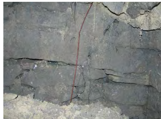
Plate 8: Northern wall 10 and fill (14).
