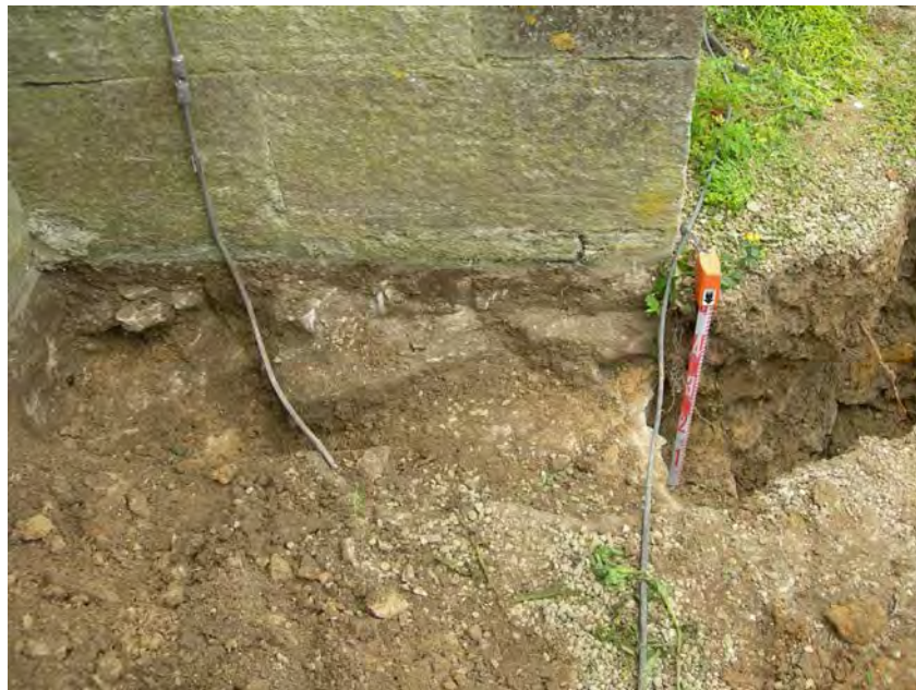
Plate 3: Foundations of Church Tower.
