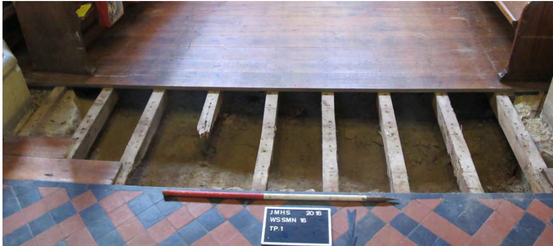
Plate 3: General view of trial hole 1
