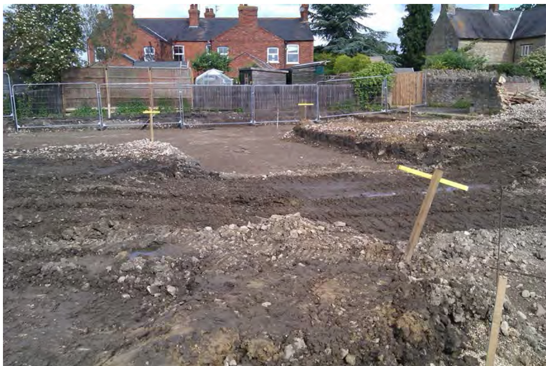
Plate 1. Unmonitored access road adjacent to Area 200
