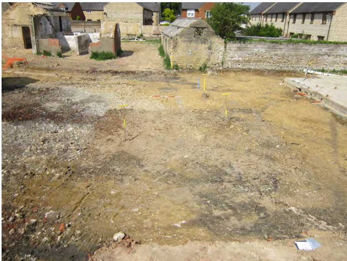
Plate 4. Area 200 (central part); looking north over crane-base; gully 2007 exiting Area 700 to east (right of picture)
