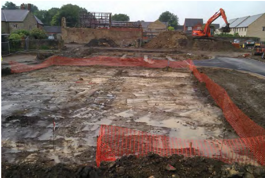
Plate 12. Area 300; looking north after cleaning, prior to excavation
