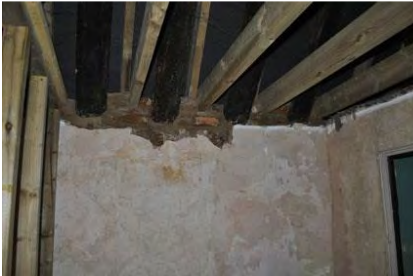
Plate 36: Rafter bases south wall
