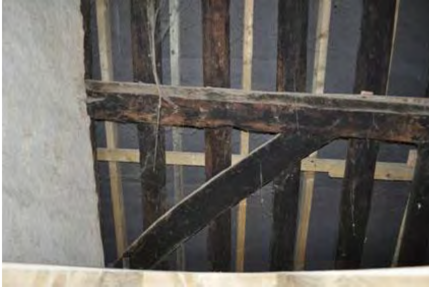
Plate 35: Wind-brace between lower purlin and wall plate
