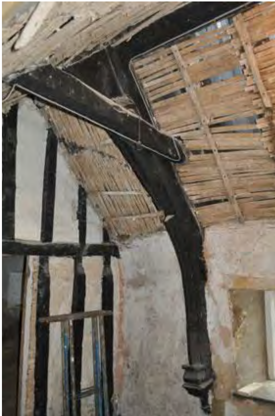
Plate 40: Base of truss against north wall
