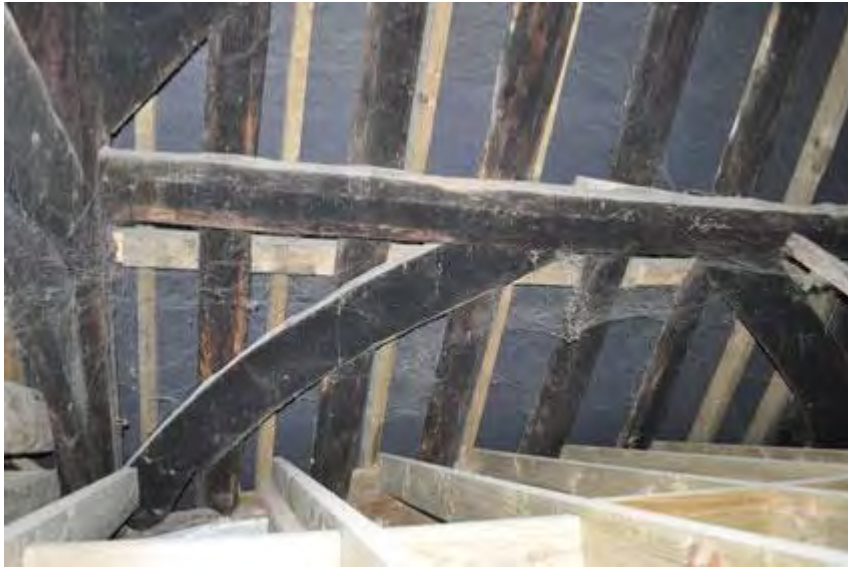
Plate 33: Wind-braces between the lower purlin and wall plate
