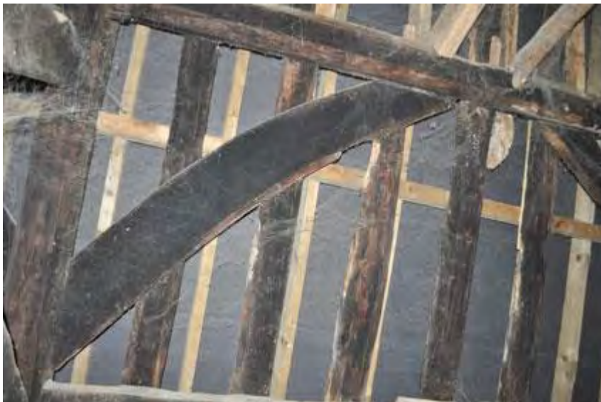
Plate 28: Wind-brace between purlins
