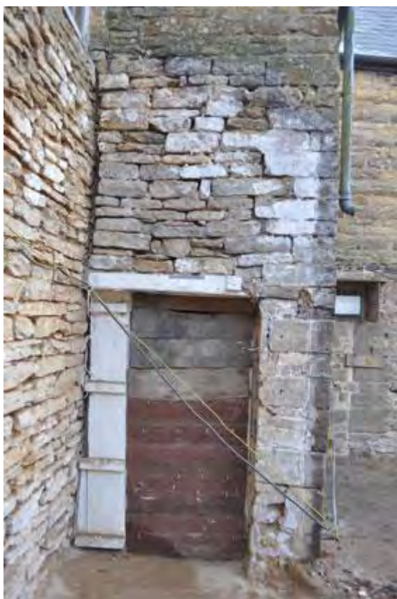
Plate 11: Butt joint in rebuild
