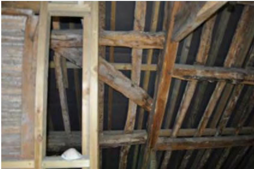
Plate 22: Wind-brace in attic S1
