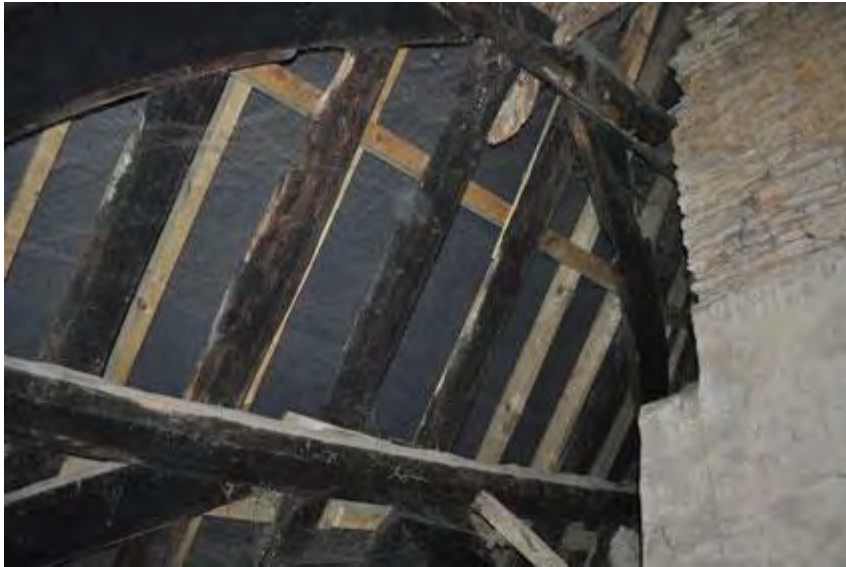
Plate 27: Wind-brace between purlins
