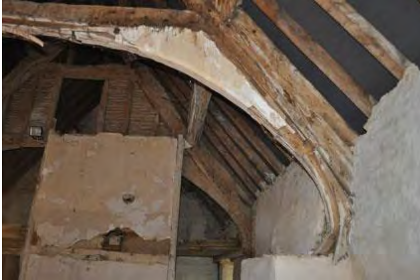
Plate 20: Lower part of truss above a wall stub
