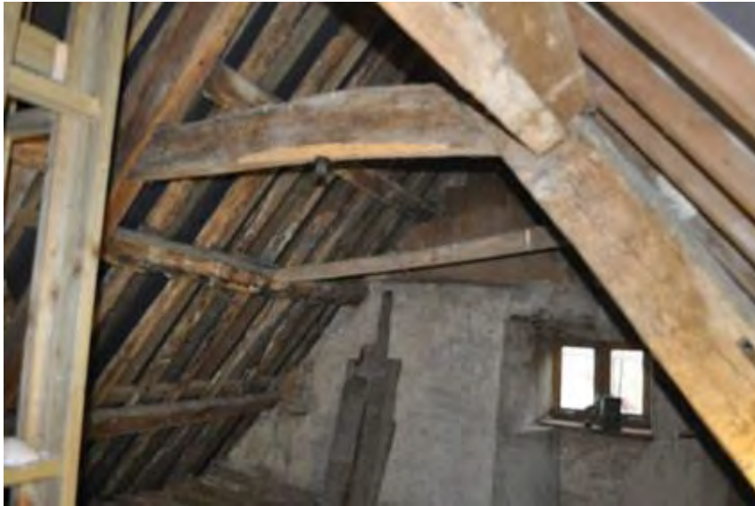
Plate 21: A frame in attic
