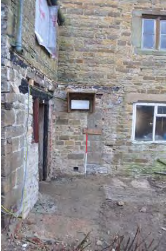
Plate 12: Blocked doorway and window
