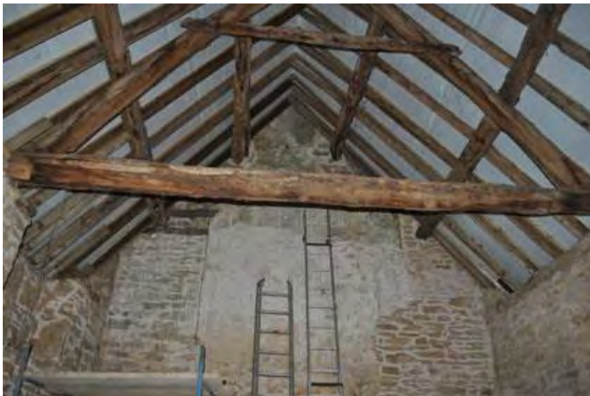
Plate 13: Blocked window in gable and in east wall
