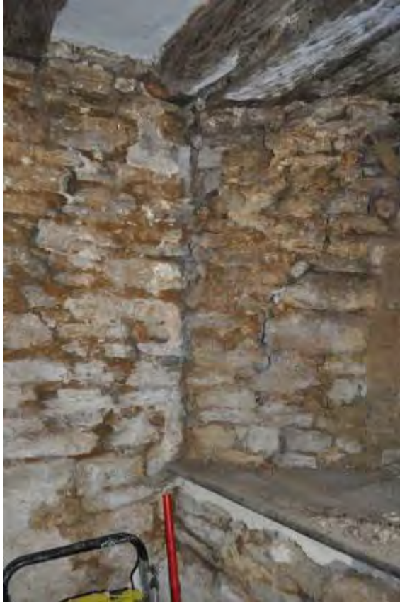
Plate 7: Butt joint adjacent to window
