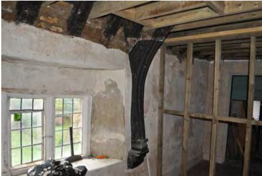
Plate 39: Base of truss against south wall
