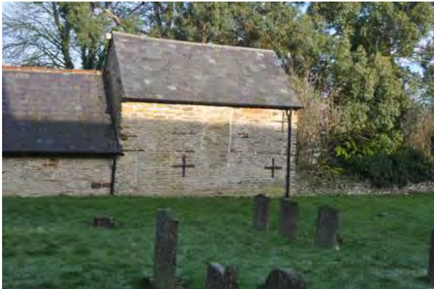
Plate 17: Butt joints and infill in the south wall
