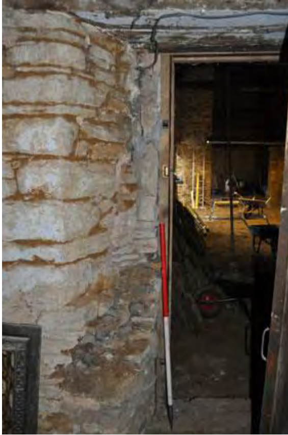
Plate 9: Door inserted in original window location
