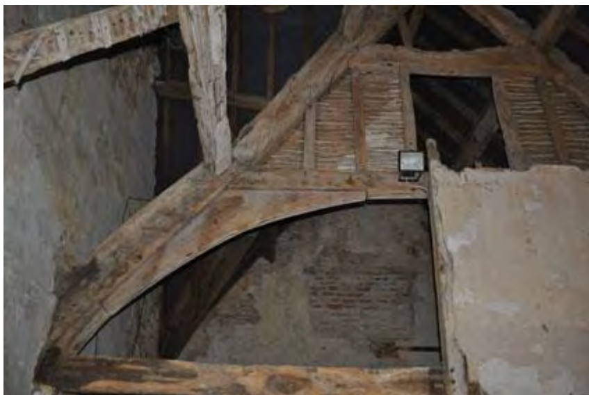
Plate 43: Truss with blocked window behind
