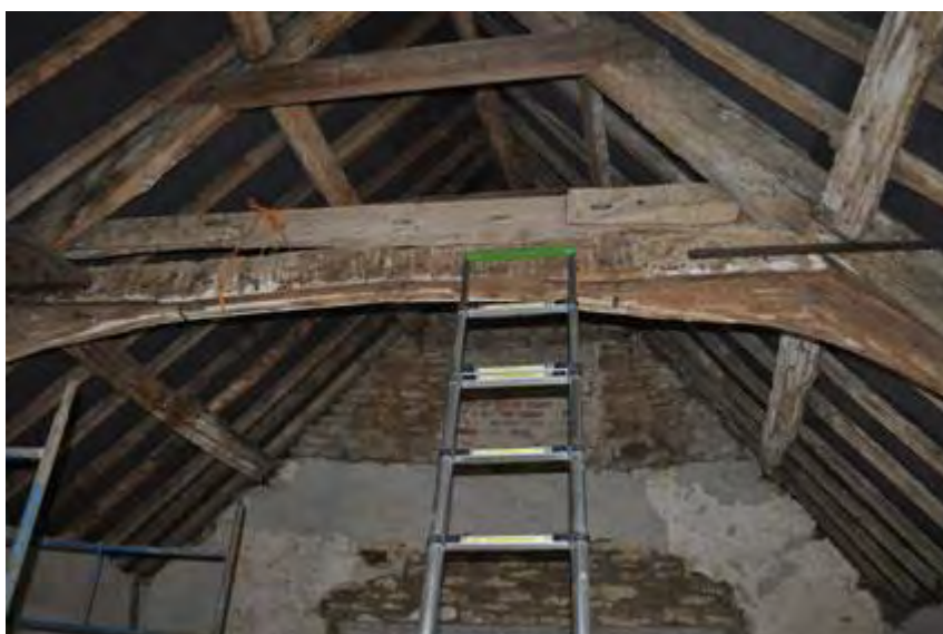
Plate 44: Truss with blocked window behind
