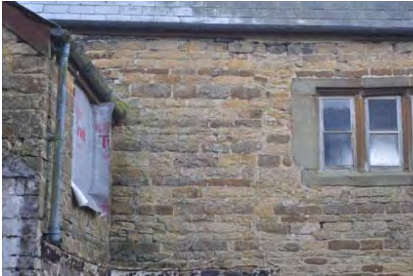
Plate 18: Blocked window F1 and F3
