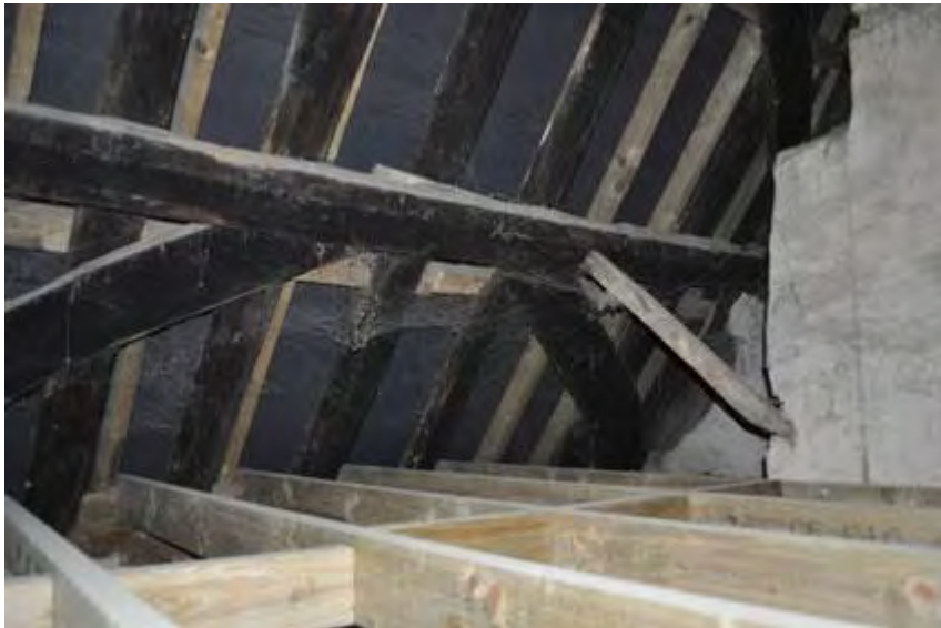
Plate 32: Wind-braces between the lower purlin and wall plate
