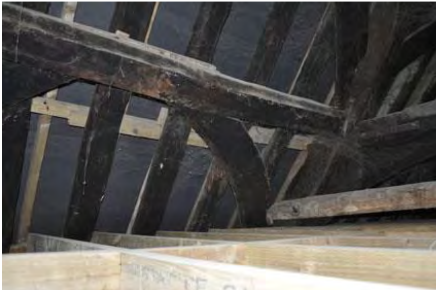
Plate 34: Wind-braces between the lower purlins and wall plate
