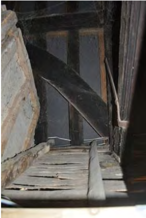
Plate 29: Wind-brace between purlins
