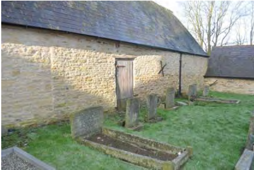
Plate 16: Butt joint in wall relating to original build
