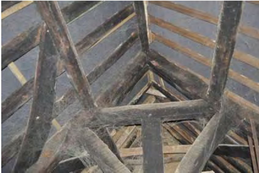
Plate 25: Ridge beam central
