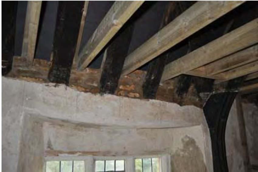
Plate 37: Rafters bases in the south wall
