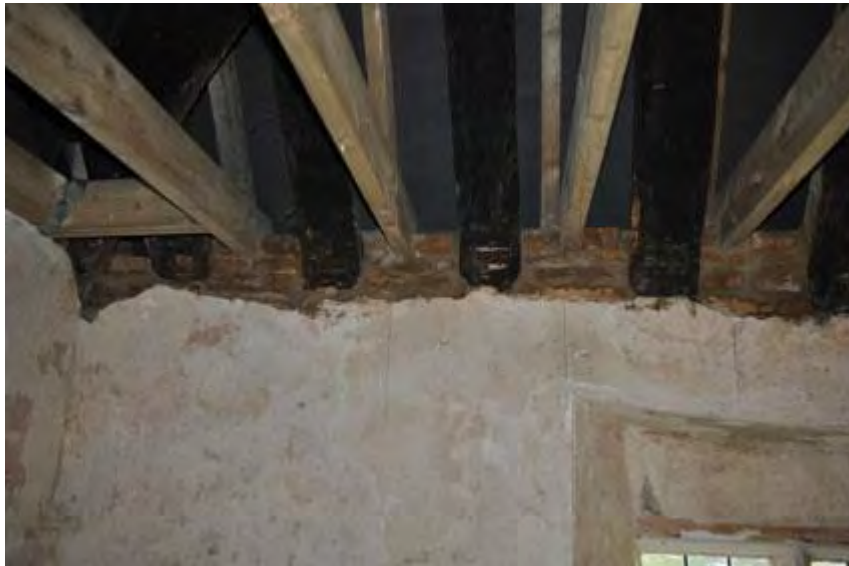
Plate 38: Rafters bases in the south wall
