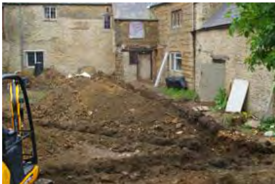
Plate 49: General shot of service trenches
