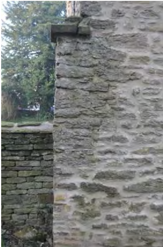
Plate 4: Reworking of building corner
