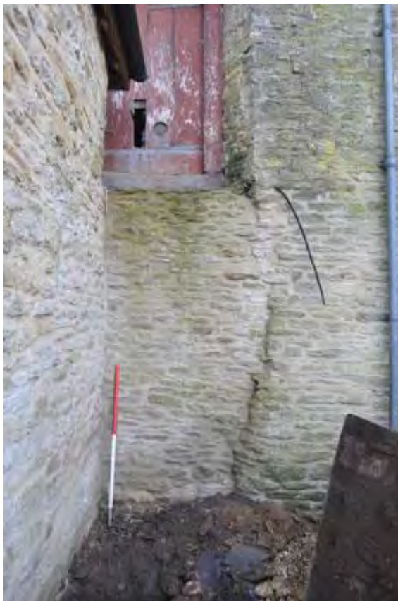
Plate 10: Reworking of the original wall
