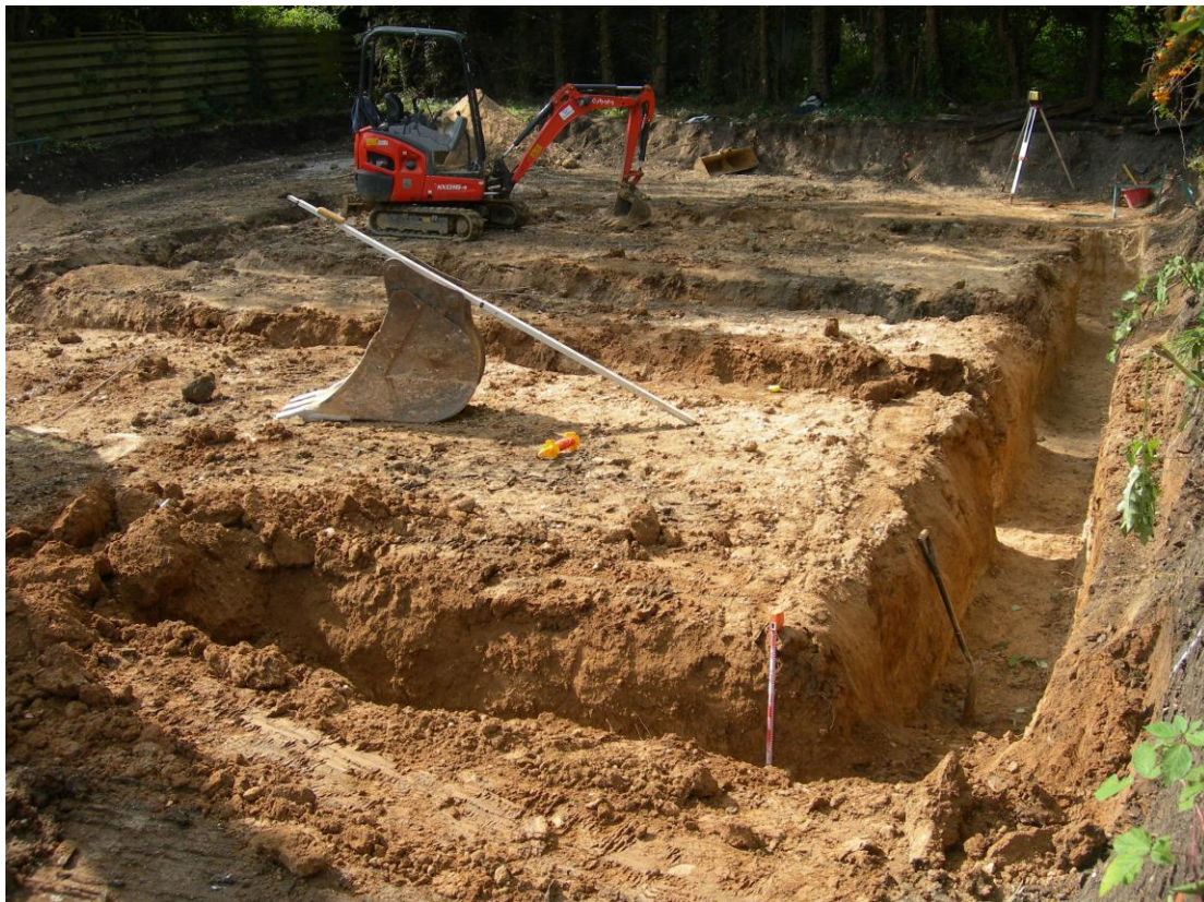
Plate 2. Foundation trench looking south.
