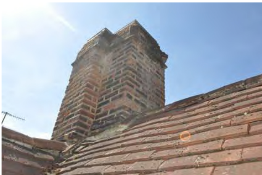
Plate 6: Northwest side of chimney
