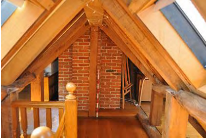
Plate 13: Chimney from north in attic
