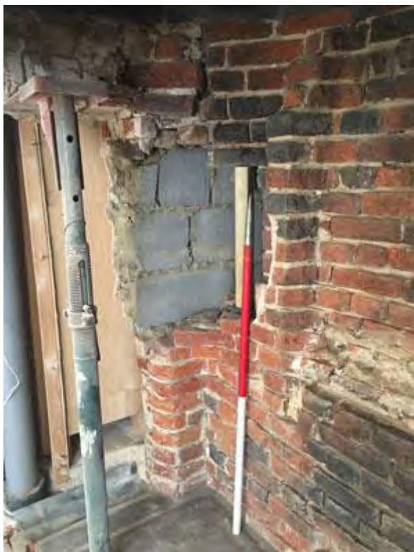
Plate 21: Line of rebuild above bread oven entrance
