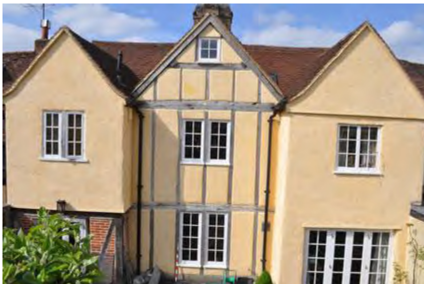
Plate 3: Rear of building
