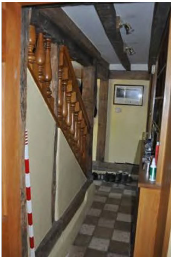
Plate 25: Passage with sill beam
