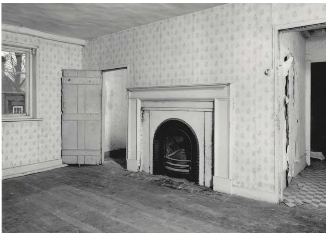
Plate 24: First floor fireplace
