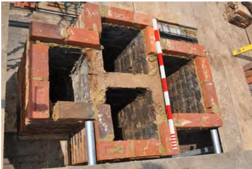
Plate 16: Top of chimneystack removed from northeast
