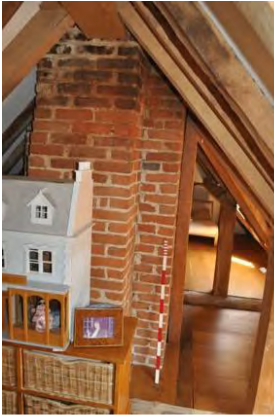
Plate 15: Chimney from east in attic
