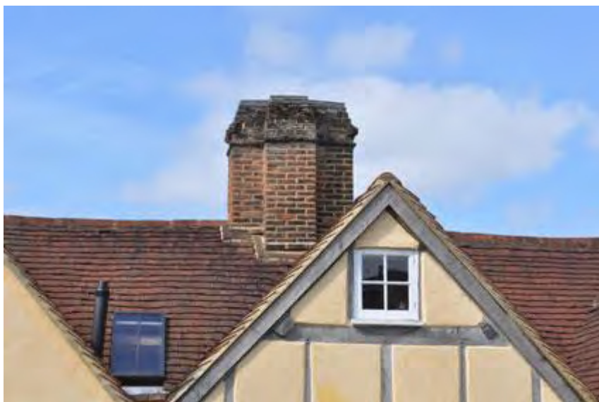
Plate 4: Rear of chimney
