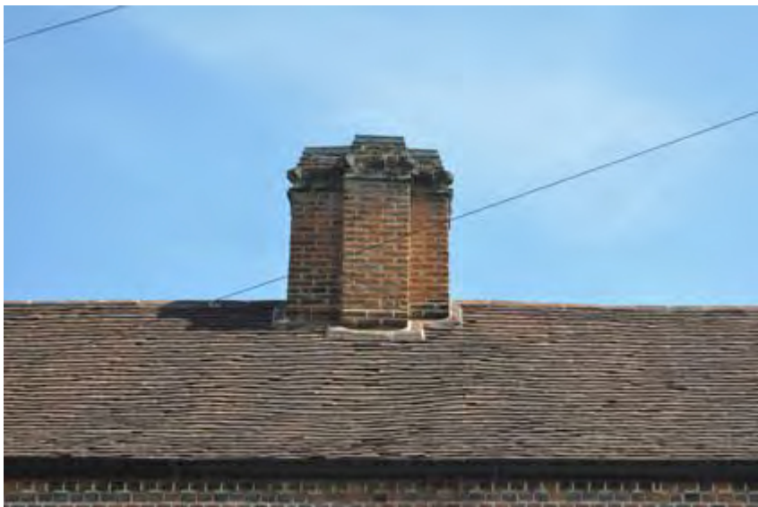
Plate 2: Chimney from front
