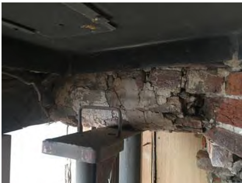
Plate 22: Area of rebuild left-hand wall
