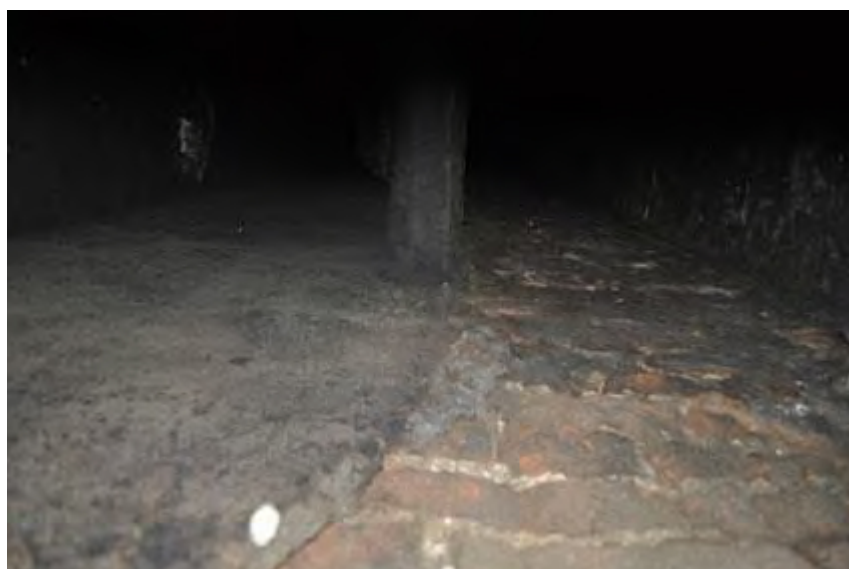
Plate 23: Internal division of chimney flue
