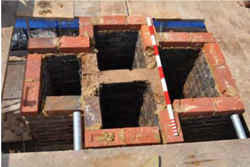
Plate 17: Top of chimneystack removed from north
