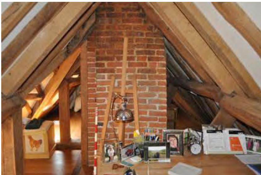
Plate 14: Chimney from west in attic
