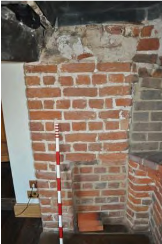
Plate 11: Reworked left-hand wall
