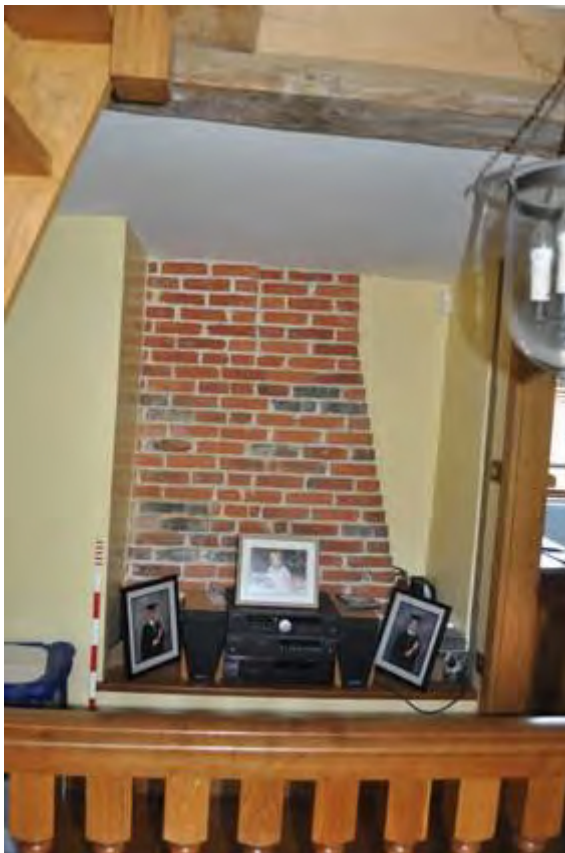
Plate 12: Chimneybreast from stairwell
