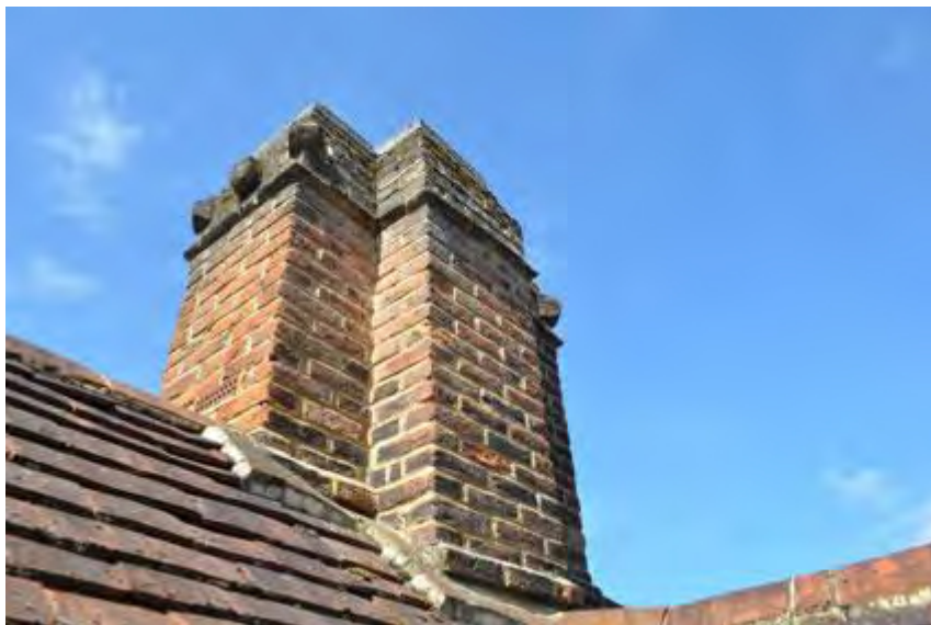
Plate 5: Northeast side of chimney
