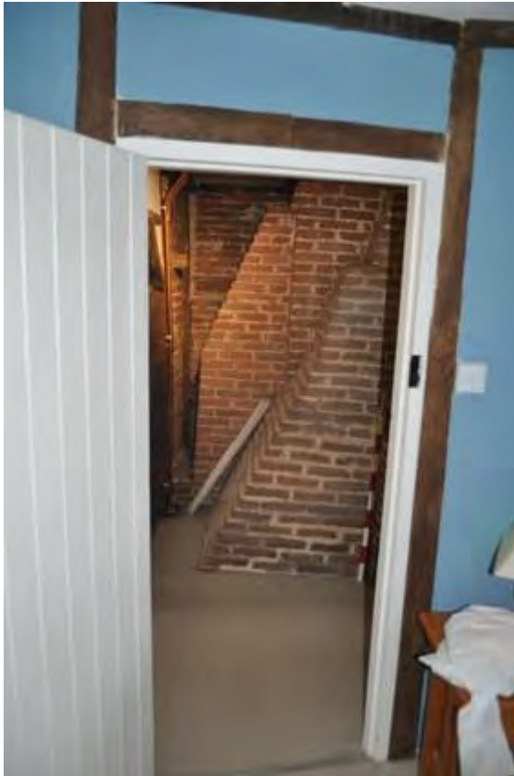
Plate 27: Dells Farmhouse chimney system
