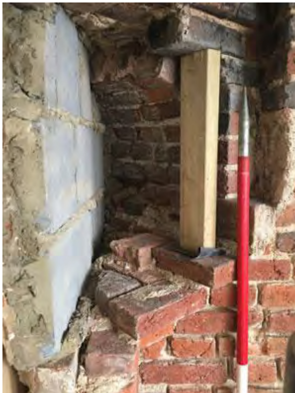
Plate 20: Opening to bread oven
