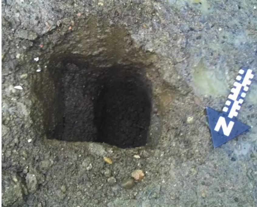
Plate 1. Post-excavation of the representative pile, S.1.
