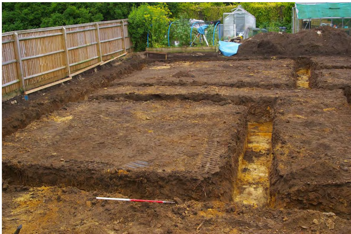
Plate 2. Foundation trench looking south
