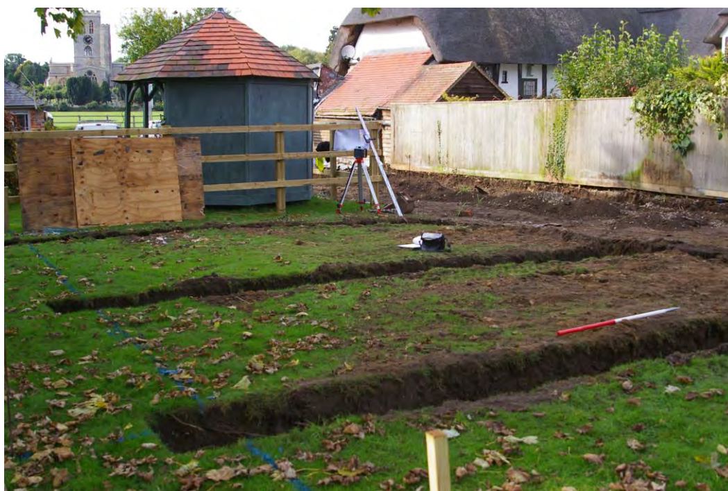
Plate1. Garage trench looking northwest
