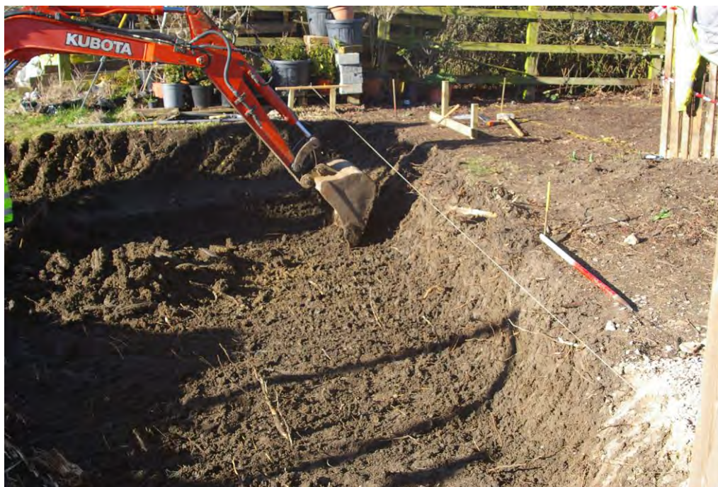
Plate 1. Working photograph of trench looking north
