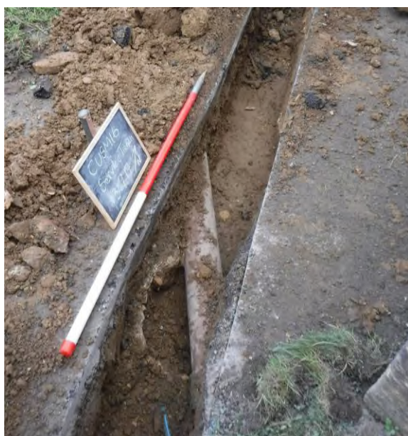
Plate 11. Area 3, general shot of Service Trench 1. W-NW view.
