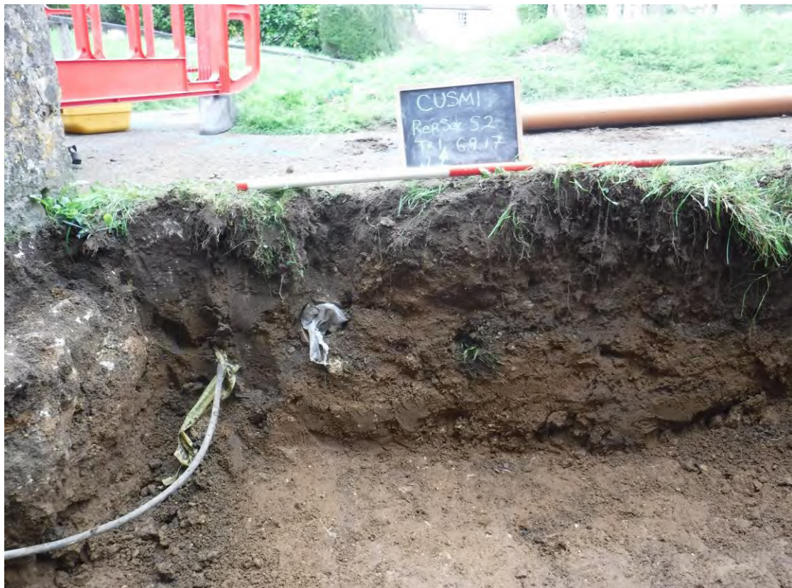
Plate 6. Area 1, Representative Section, S2. North view. (Note: Ceramic drain for soakaway seen covered in plastic - to the right of the electric cable - and gravel drain seen directly below sign-board and to the right of the ceramic drain).
