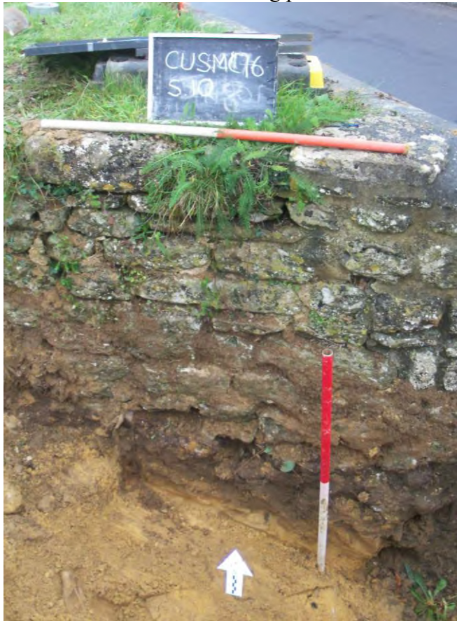
Plate 16. Area 5, S.10. North view.
