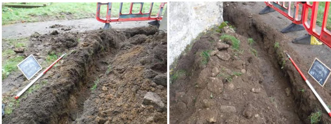
Plate 8 & 9. Area 2, general shot of Service Trench 2. North & west views respectively.
