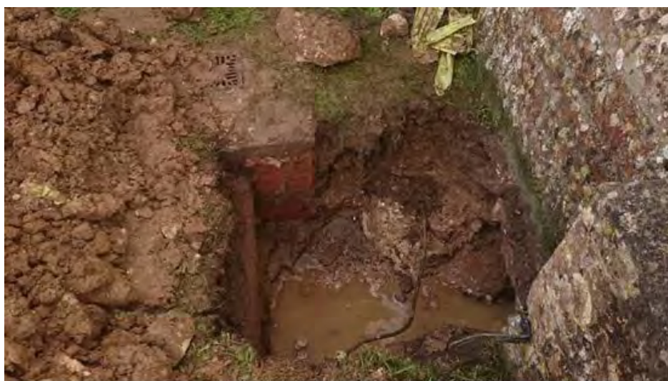
Plate 1. Test pit 1. South view.
