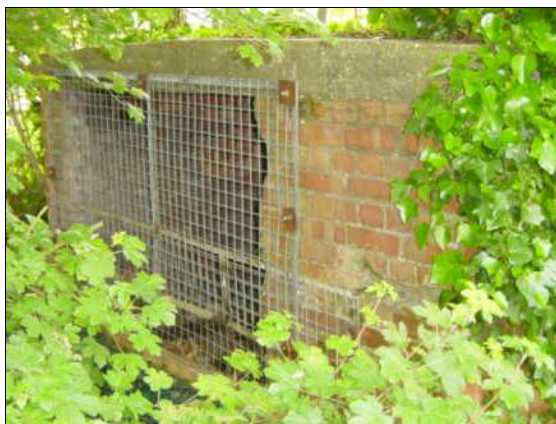
Plate 3: External view of the inaccessible eastern end of the shelter (B8).
