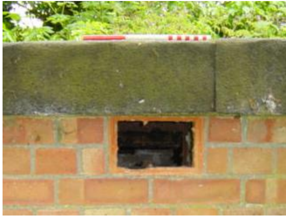
Plate 6a: Remains of broken - through ventilation brick
