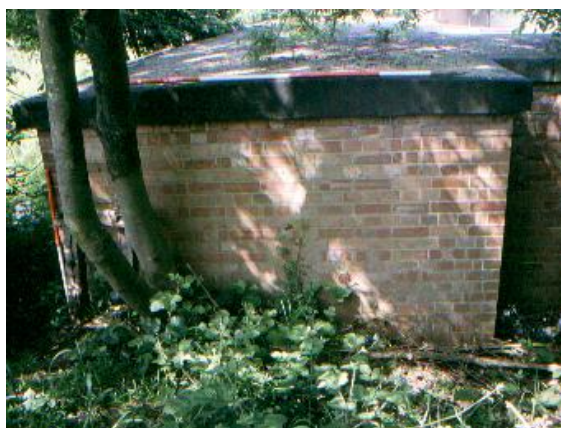
Plate 1: Detail of construction materials
