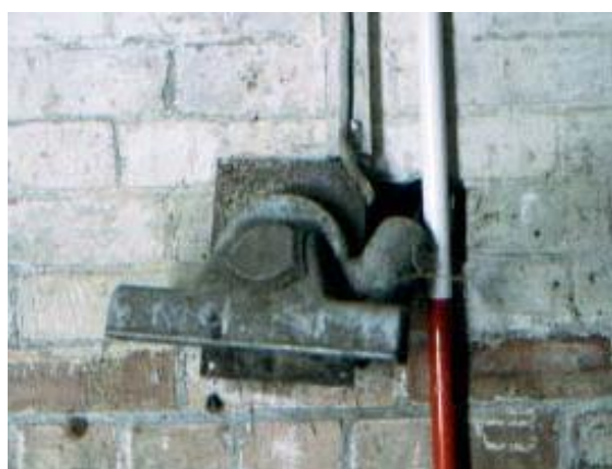
Plate 13: Extractor made from vacuum cleaner head
