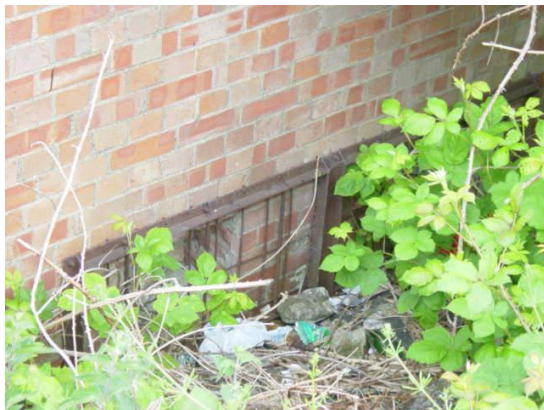
Plate 6c: Grille in situ taken from roof of adjacent western block
