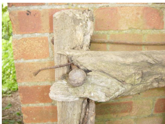
Plate 5b: Detail of bolt from front
