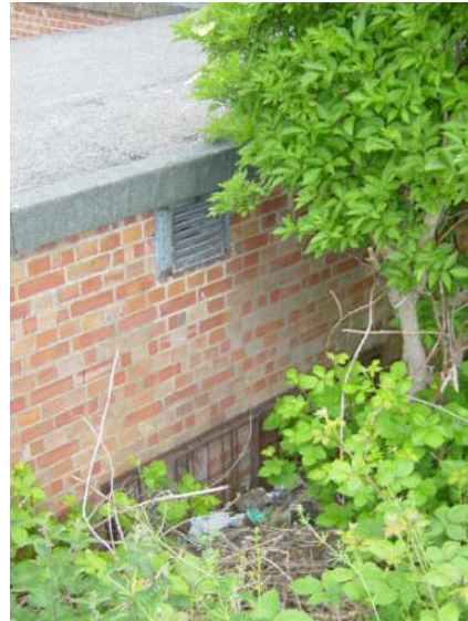
Plate 6b: Metal louver over vent and grille covering two blocked openings
