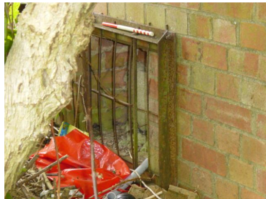
Plate 6d: Detail of eastern grille with cement blocking
