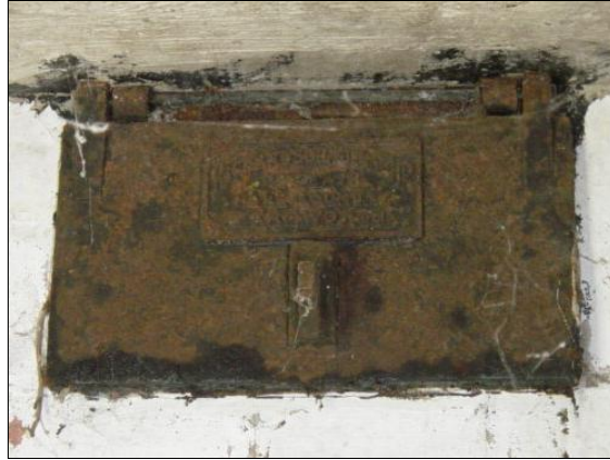
Plate 9: Closed vent in interior
