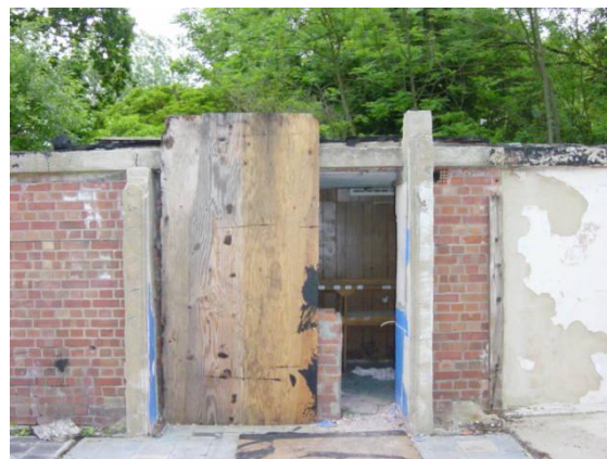
Plate 8: Modifications to create bar and access
