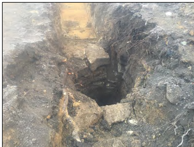
Plate 13: General view of well. North West facing
