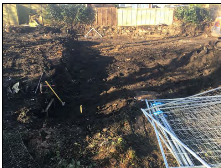
Plate 2: West facing view of the reduced construction area
