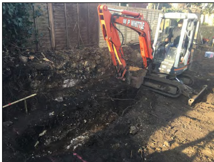
Plate 3: North-West facing view of initial trenching
