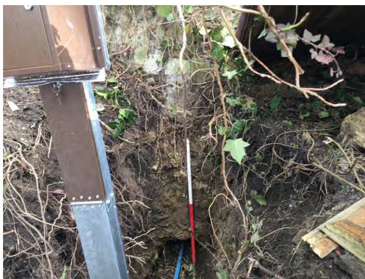
Plate 6: West facing section of cable duct
