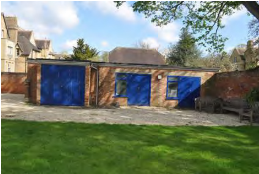
Plate 9: South elevation of garage
