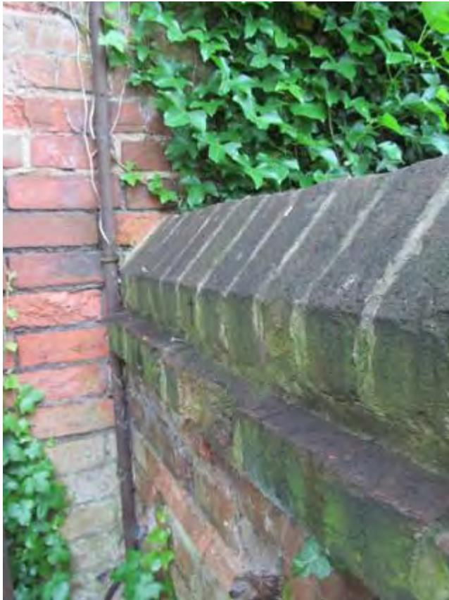
Plate 15: Joint between Wall 1 and Wall 4
