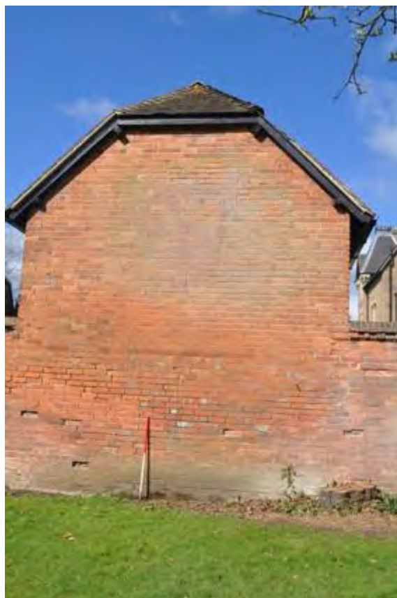
Plate 1: East elevation of Coach House
