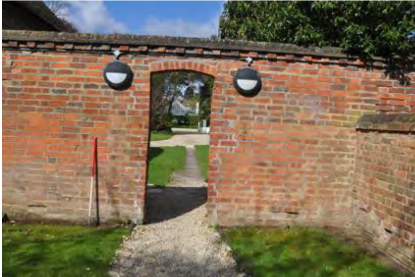
Plate 12: North entrance in Wall 1 (view to west)
