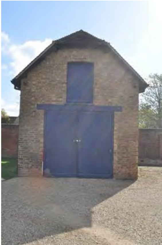
Plate 3: West elevation of Coach House
