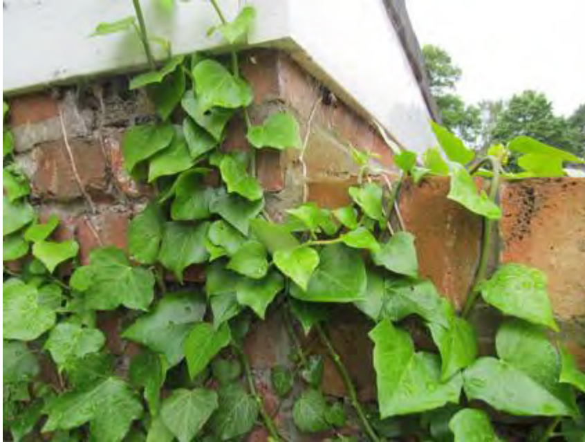
Plate 8: Top of north edge of east elevation
