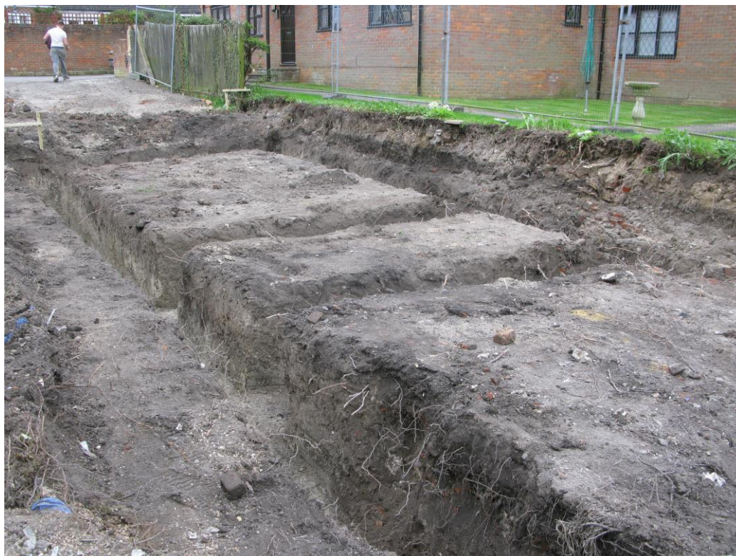
Plate. 1 Foundation trench looking southeast
